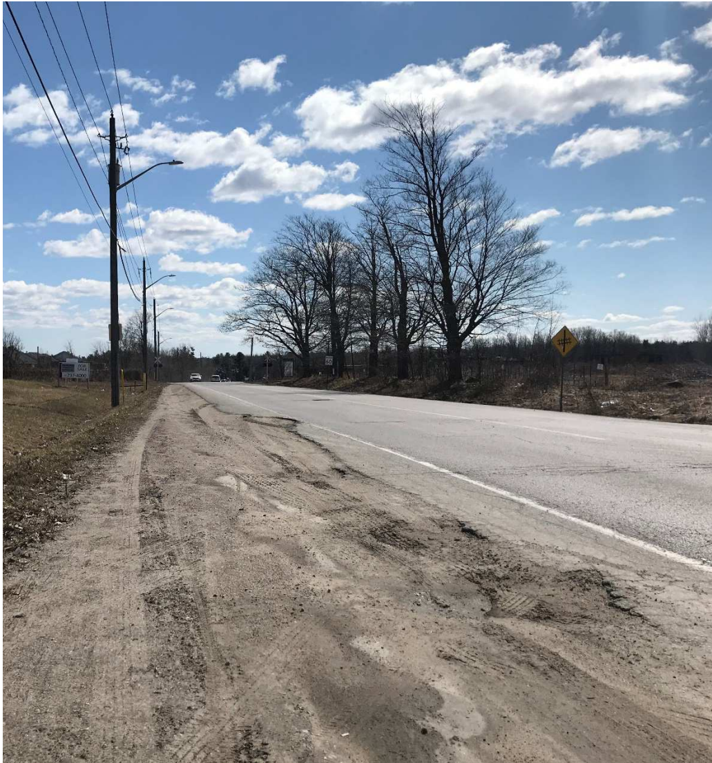
Picture taken from Site Access facing South on Huronia Road
