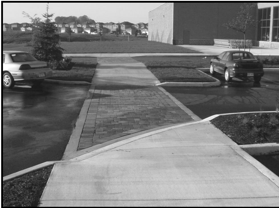
This pedestrian route is clearly defined through the use of contrasting surfaces.
