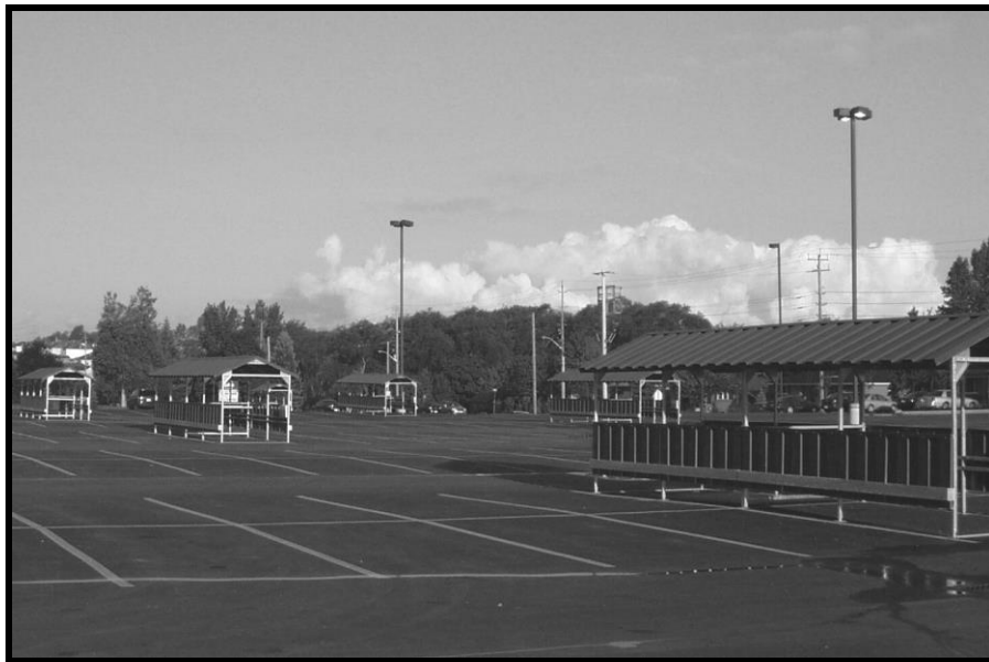
Shopping cart corals are distributed throughout the parking area.
