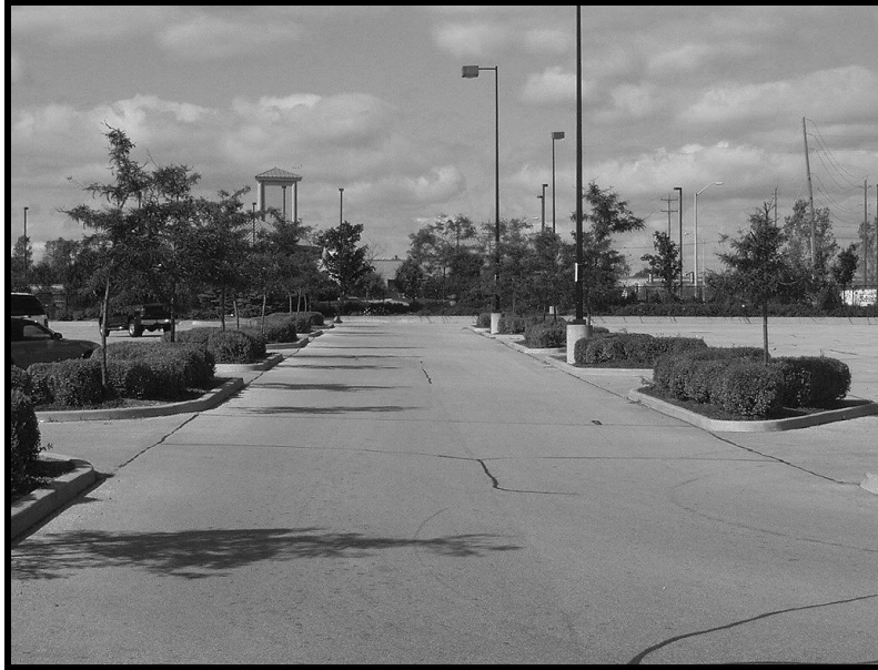
Landscaped traffic islands break up large parking areas and help delineate primary vehicle routes.
