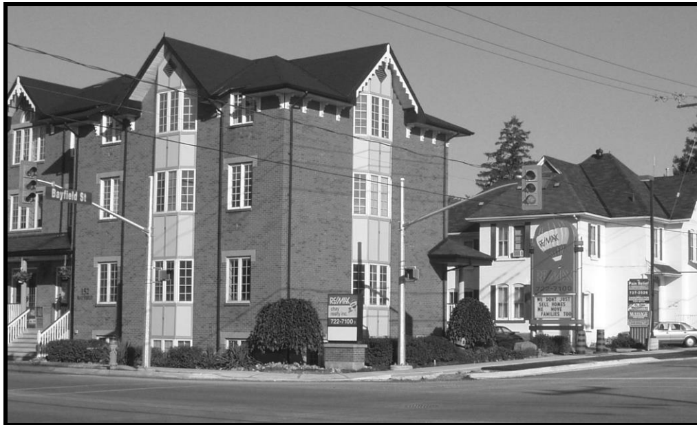
This newer office development is consistent in design and scale with the neighbouring area.
