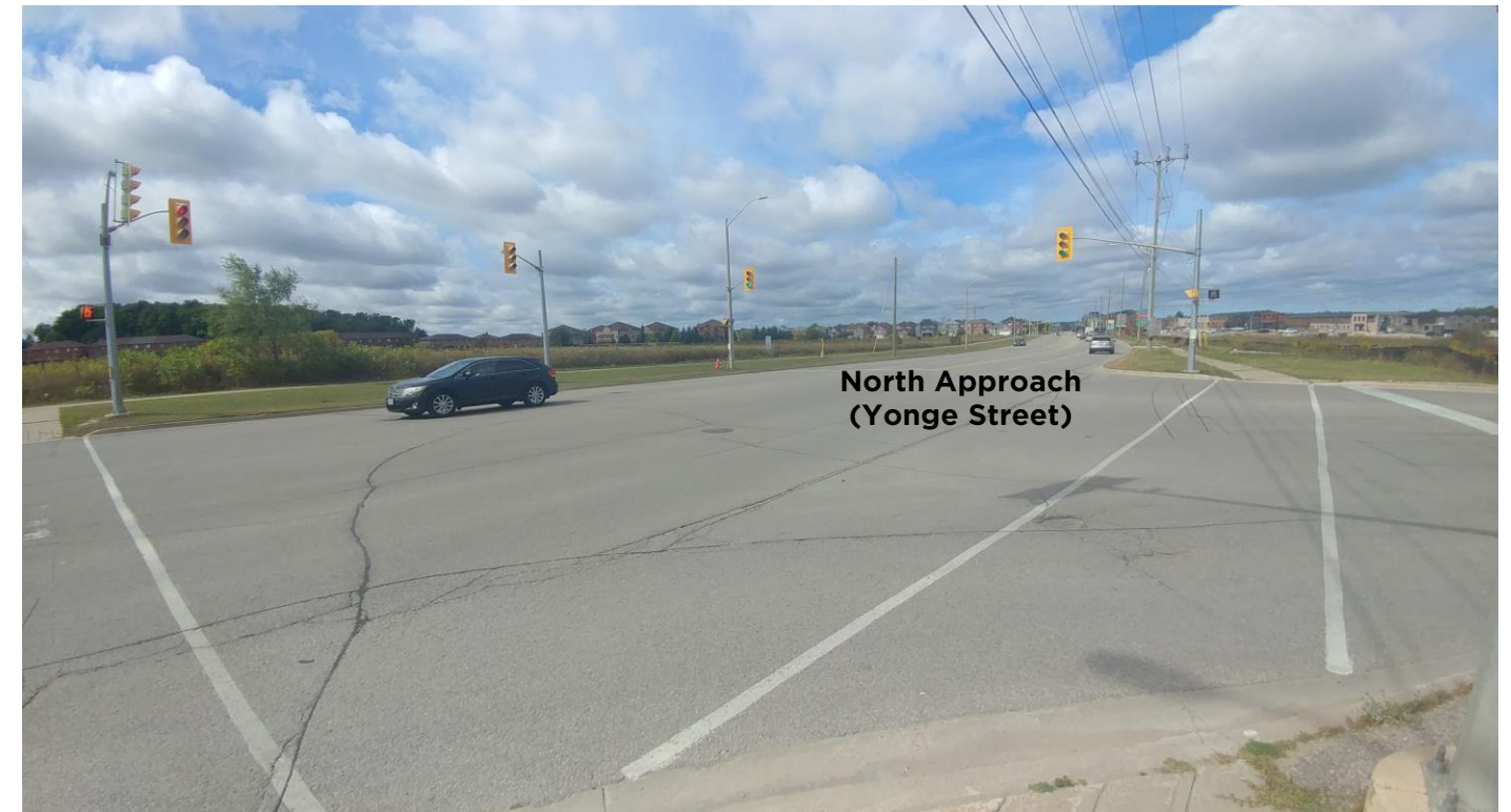
Intersection of Yonge Street & Barrie South GO access - north approach
