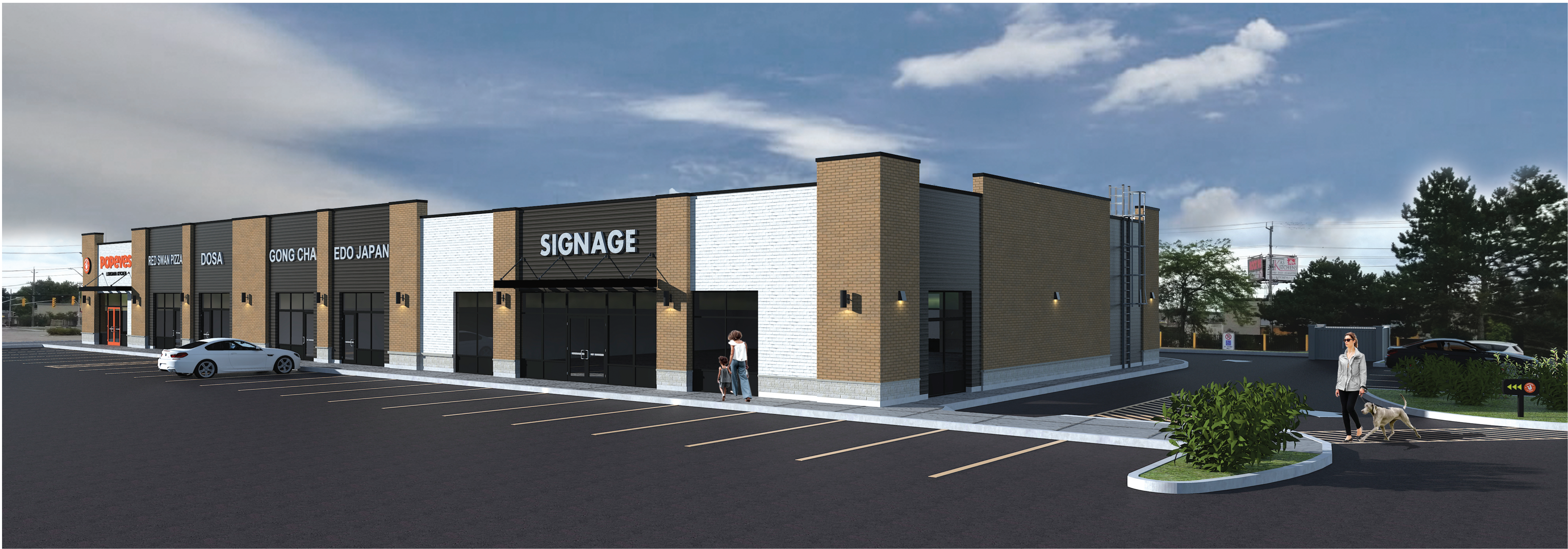
WEST VIEW FROM PARKING LOT
