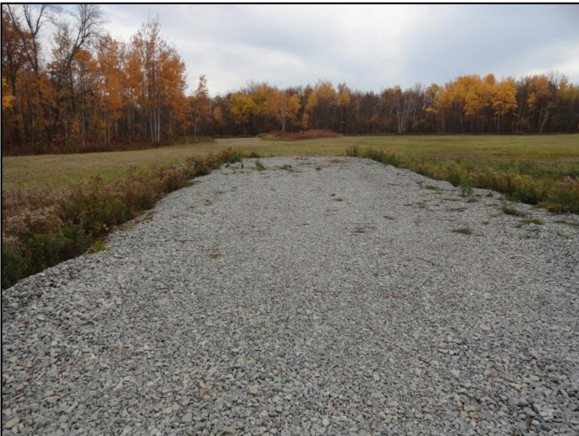
Photograph 3. Southward view of current access to CUM1-1-A at 259 Salem Road (Watersand Construction Inc.) on west side of the property
