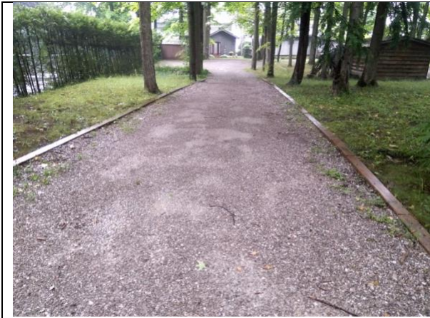
IMAGE 1 VIEW OF GRAVEL DRIVEWAY
