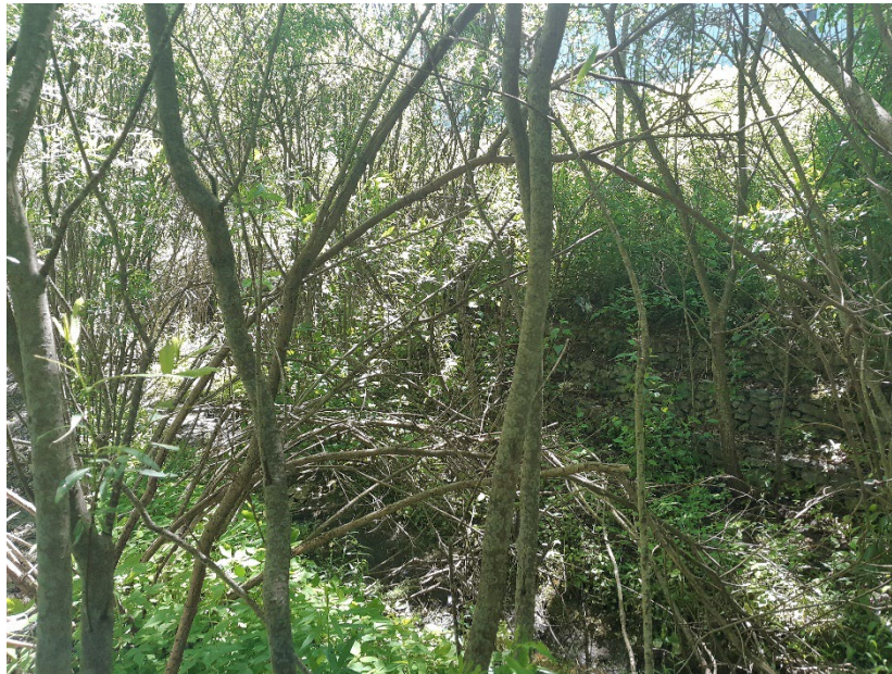
Photo 18 Reach B showing channel banks lined with gabion baskets, June 7, 2021.
