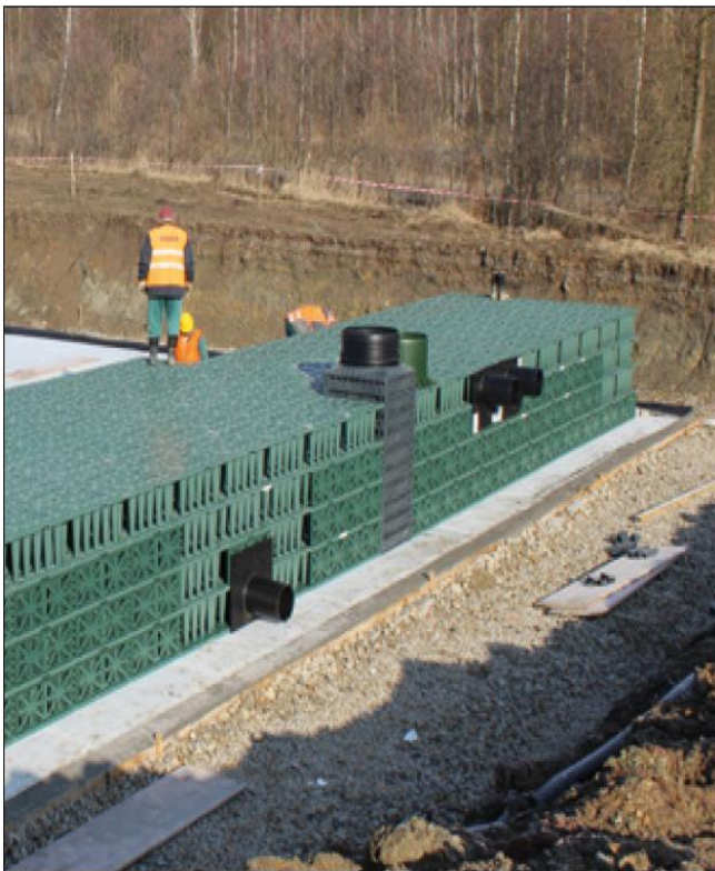
FIG#3: PIPE ADAPTER INSTALLATION
