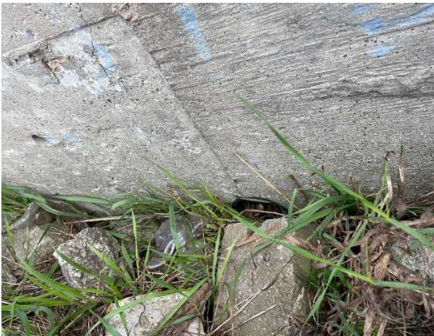
75mm diameter orifice tube on the SWM Outlet Control Structure
