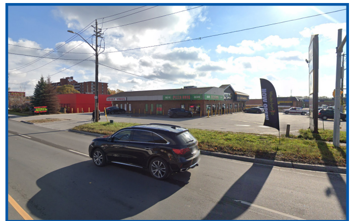
Figure 2.0n - Commercial plaza at 285 Dunlop St. W.
