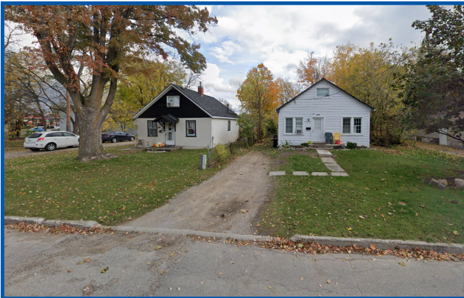
Figure 2.0e - Subject site as viewed from Henry Street looking south, 119 and 121 Henry Street
