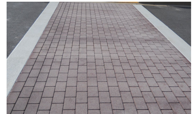
IMPRESSED ASPHALT CROSSWALK
