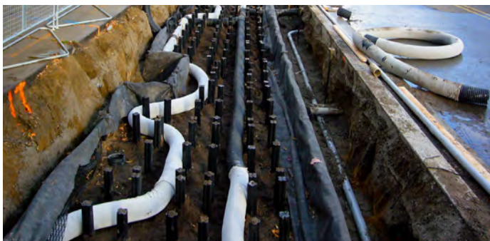
Figure 4. Distribution pipe on top of soil (image courtesy of City of Toronto)
