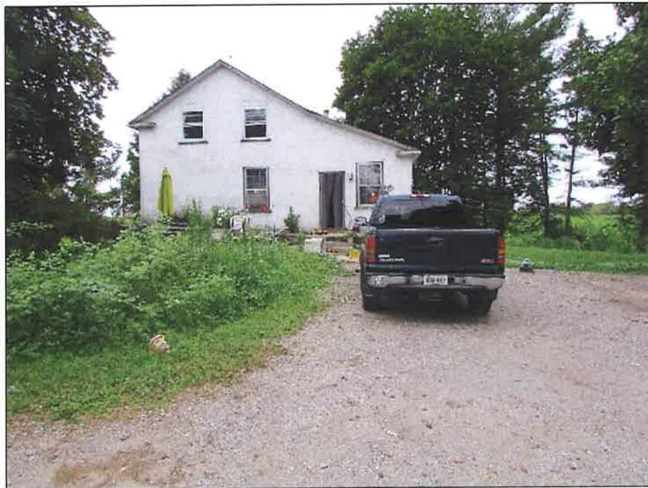
General view of the residential building in the southern section of the subject site (facing west)
