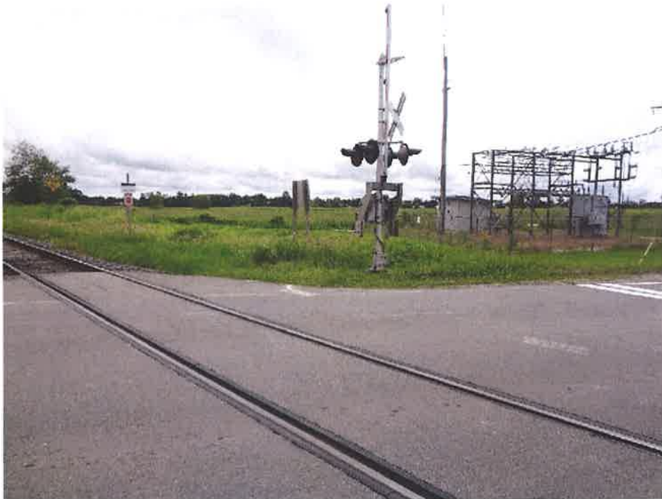
General view of the railway tracks and transformer station to the west and southwest of the subject site, respectively.
