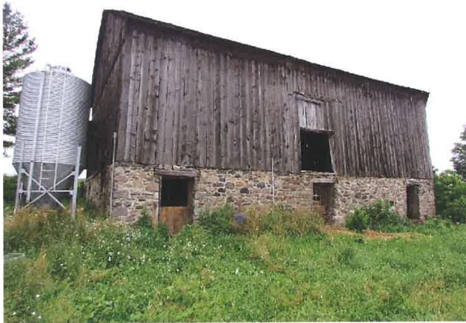
General view of the barn on the southern section of the subject site.
