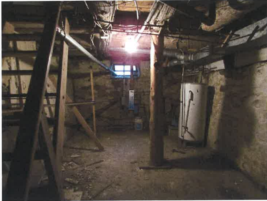
General view of the basement of the residential building.
