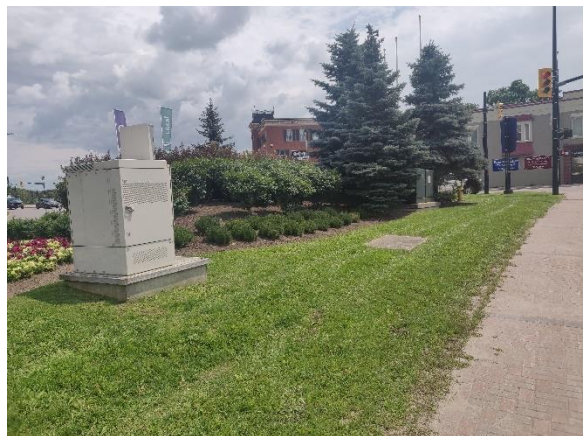
Image 16: Utilities present in island median; no potential
