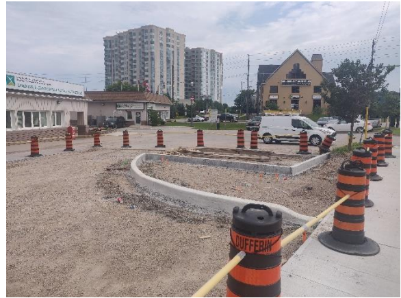
Image 31: Disturbed Bradford Street right-of-way and 19 Bradford Street; no potential
