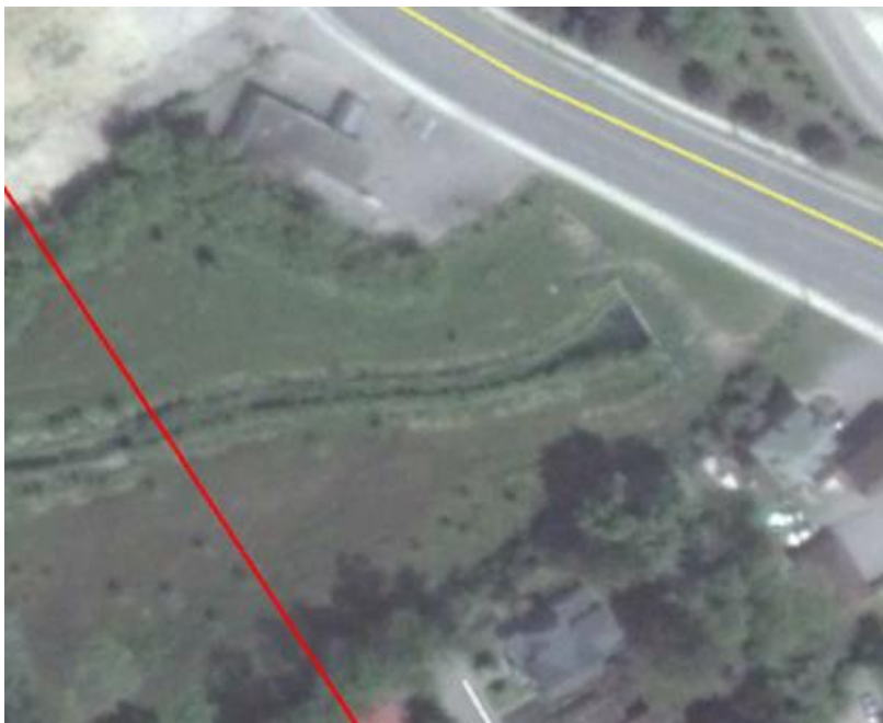
Image 48: Conditions of 240 Bradford Street during June 2013 showing demolition and channelization disturbance; no potential
