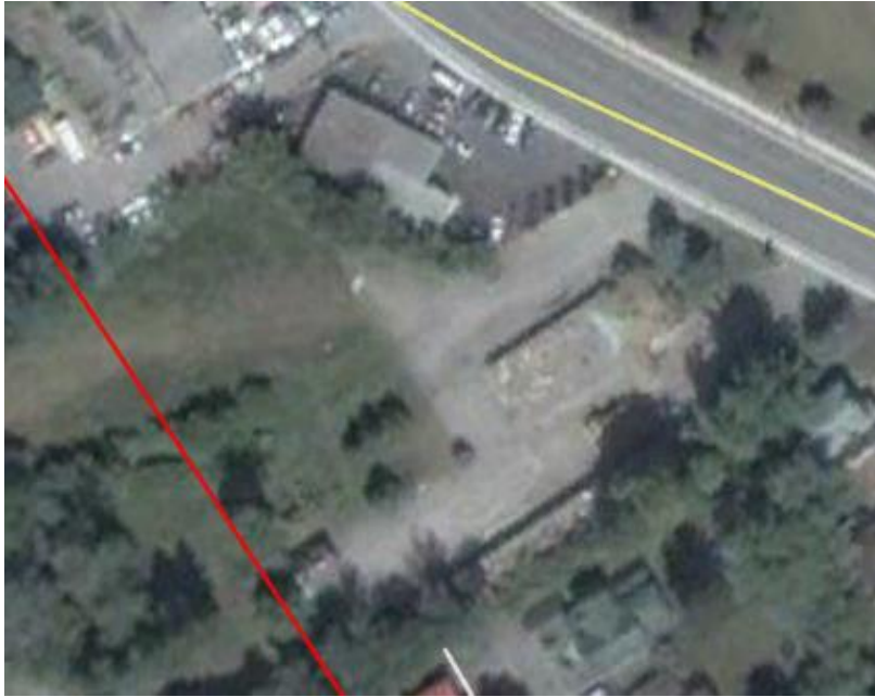
Image 47: Conditions of 240 Bradford Street during August 2006
