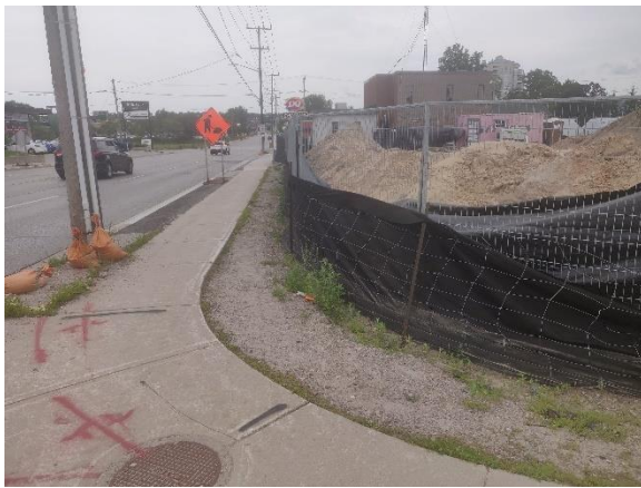
Image 25: Disturbed Bradford Street right-of-way and 111 Bradford Street; no potential
