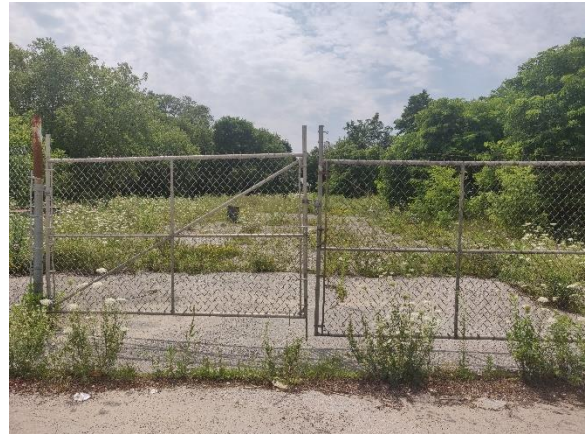
Image 19: Demolition disturbance of 220 Bradford Street; no potential
