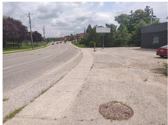
Image 20: Disturbed Bradford Street right-of-way; no potential
