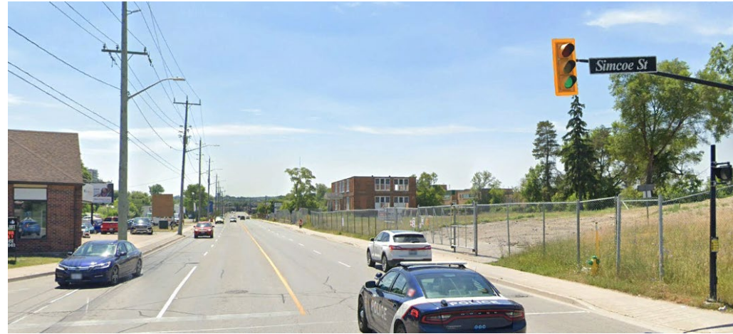
Bradford Street at Simcoe Street, looking south
