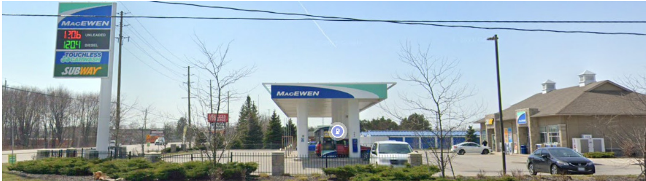
Service Station at the Northwest Corner of Miller Drive and Dunlop Street West
