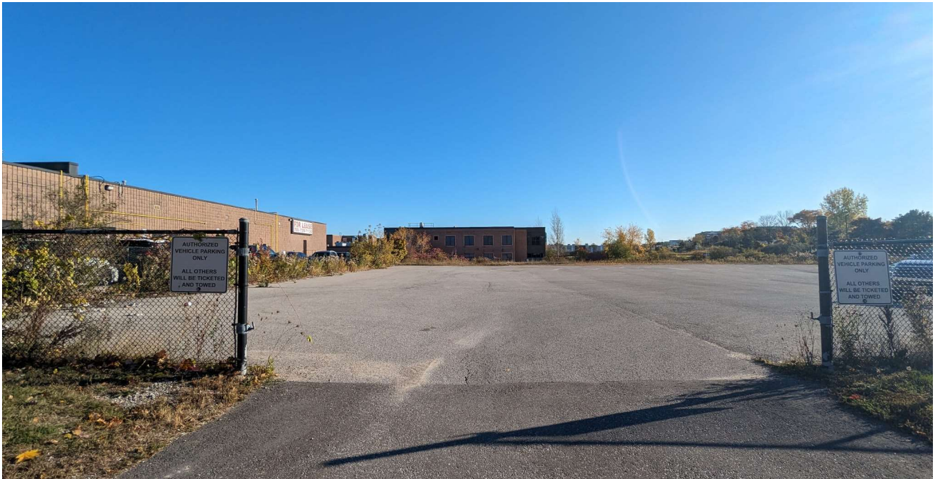
1. Front view of the northern portion of the Phase One Property, facing northeast
