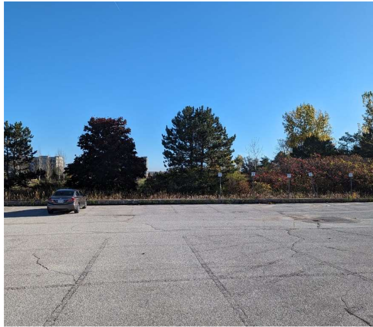
9. View of east parking lot, facing northeast
