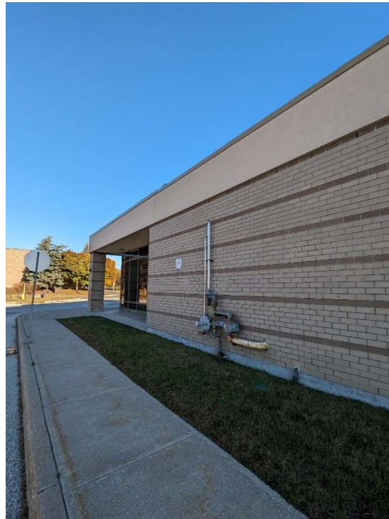
11. West side of the building, facing north
