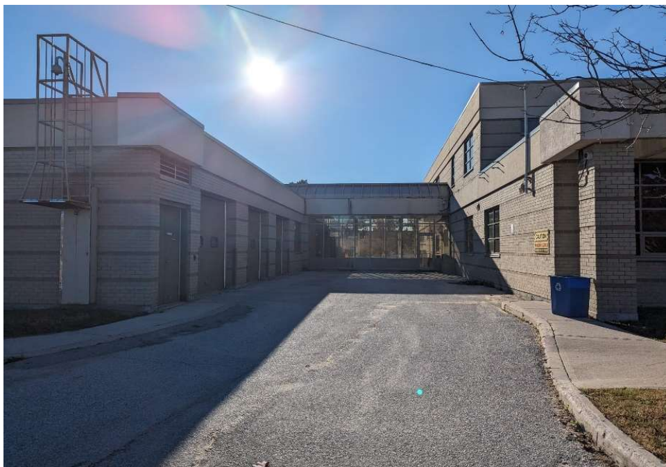
7. Front view of east portion of the building, facing southeast
