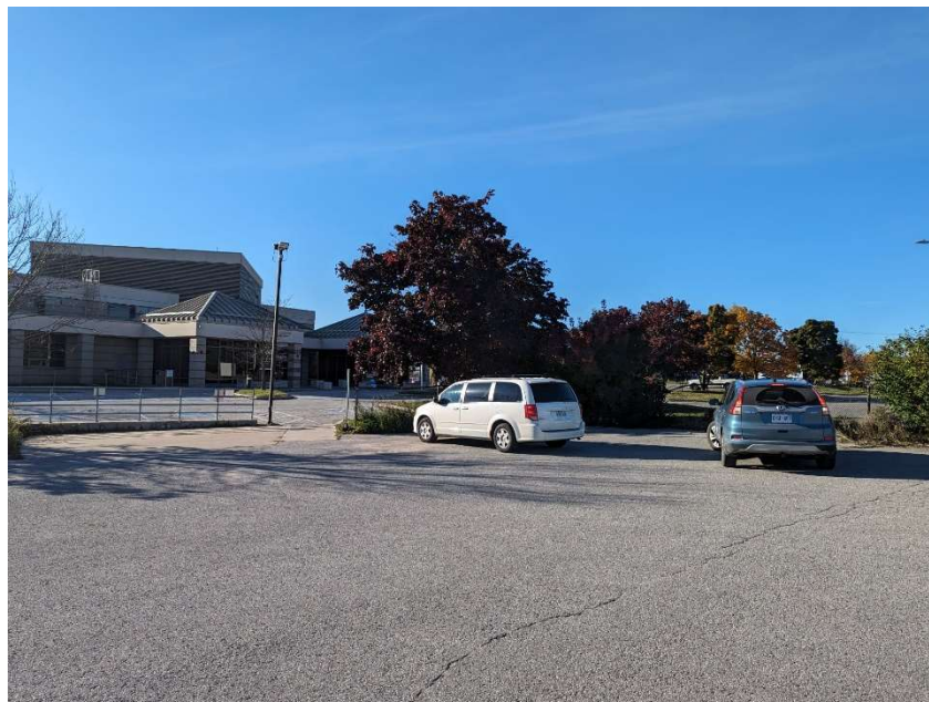
4. Access from the north portion of the Phase One Property to the south portion, facing south
