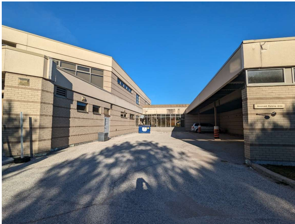
10. Reserved parking area, facing northwest
