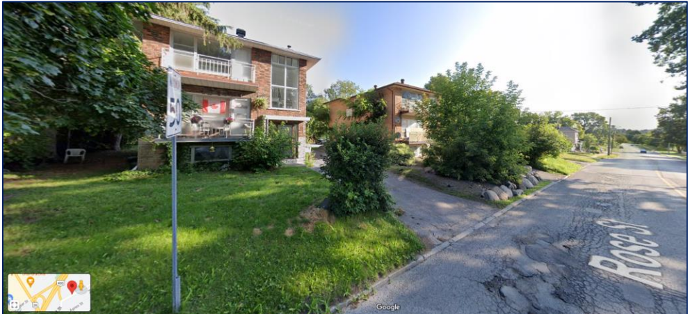
Figure 4: Rose Street - multi-unit residential, looking north west
