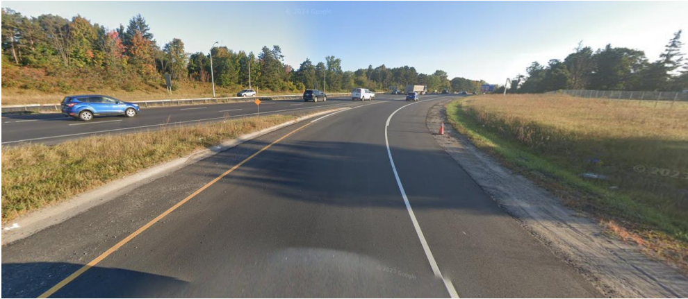
Figure 5: On ramp - Highway 400 North - controlled access transportation corridor, looking northeast
