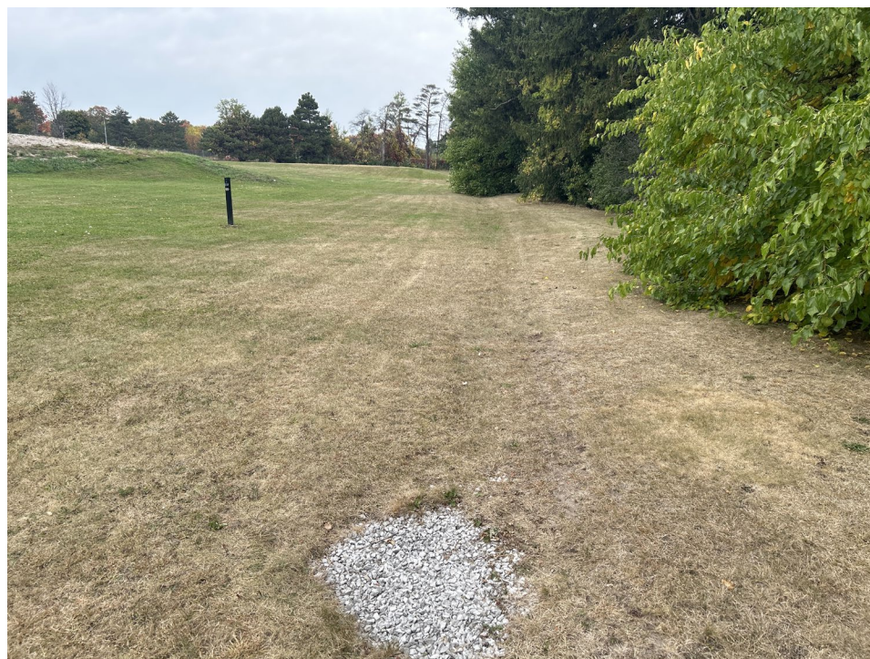
Photo 8 Gravel drainage for swale, October 2023.
