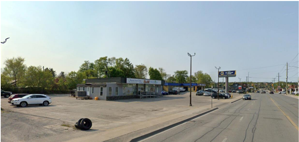
View of the Development site looking northwest from Bradford Street
