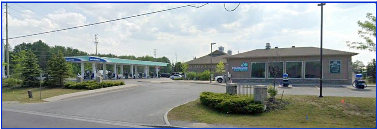
Figure 3-11 Gas Bar & Convenience Store of MacEwen Gas Station
