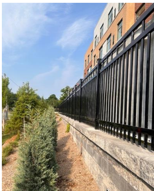
Figure 12: Retaining wall and ornamental fencing, SCHC - Orillia
