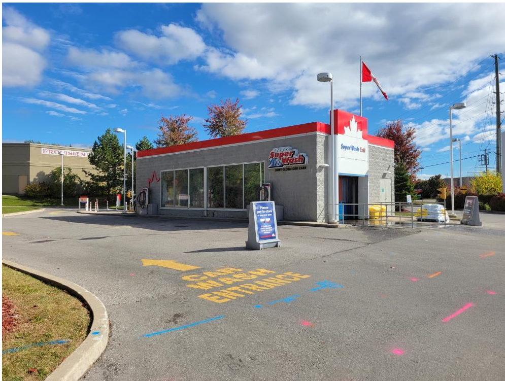
#2 General view of the carwash, looking south of the Site.
