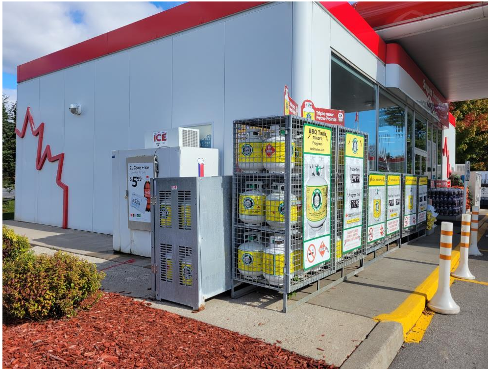
#3 View of the exterior of the convenience store, looking east of the site.
