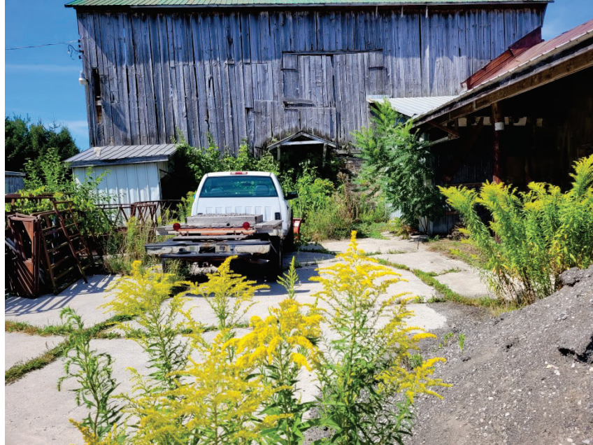
Photograph 3: View of barn on adjacent southern Phase 3 lands, facing west (August 18, 2022).
