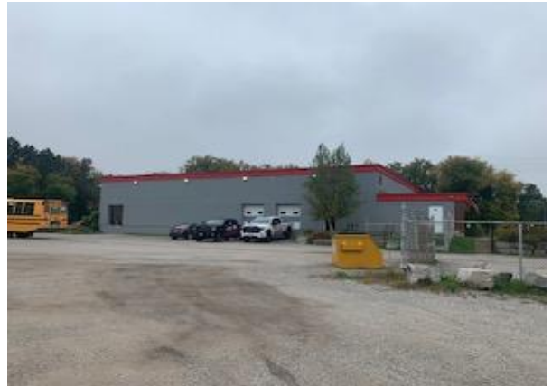
Picture 2: View of Building A, used for commercial purposes, facing west.
