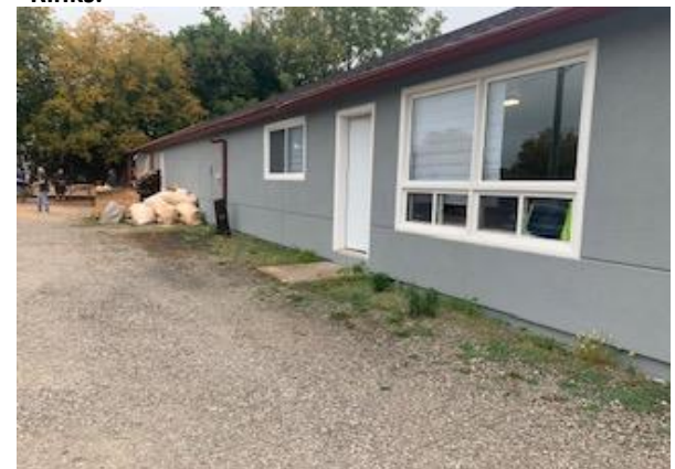
Picture 6: View of the north entrance of Site Building B, facing east.
