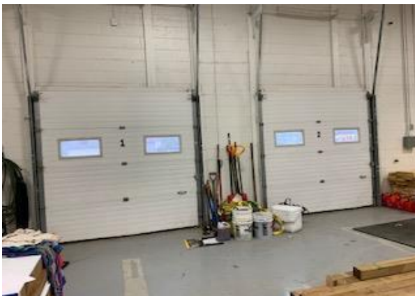
Picture 5: View of bay doors located at south end of Site Building A.
