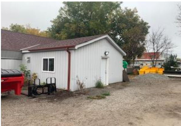
Picture 9: View of southern exterior of Site Building B, where the former AST was historically located, facing east.
