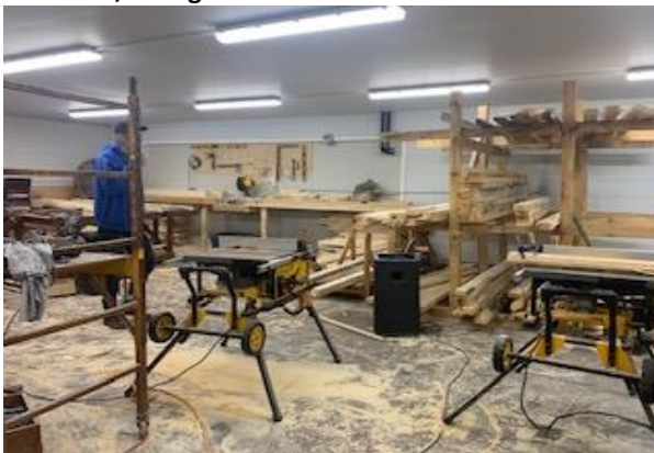
Picture 11: View of workshop in the interior of Site Building B, occupied by Cara Panel Systems.
