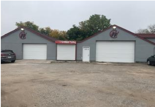
Picture 7: View of western façade of Site Building B, facing east.
