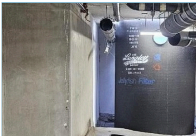
A Jellyfish Filter provides treatment to high rise tower before detention storage or water re-use in British Columbia, Canada.
