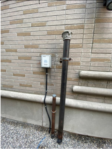
Photo 7: Vent and fill pipes associated with a AST/UST at 35-38 Hayden Street.
