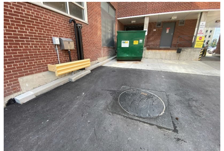
Photo 6: One set of vent and fill pipes in addition to an observation port associated with USTs at 650 Church Street.
