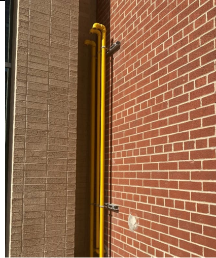
Photo 8: Vent and fill pipes associated with a UST/AST at 650 Church Street.
