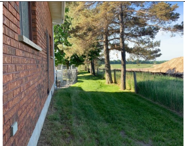
IMAGE 12 WEST SIDE OF RESIDENTIAL STRUCTURE
