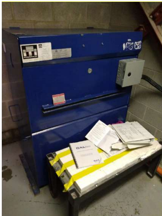
Photograph 4: elevator soil storage tank
