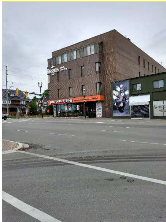
Photograph 1: view of the building, looking northwest across Dunlop Street West
