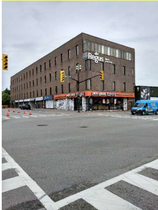
Photograph 3: view of the building, looking northeast from the High Street / Dunlop Street West intersection
