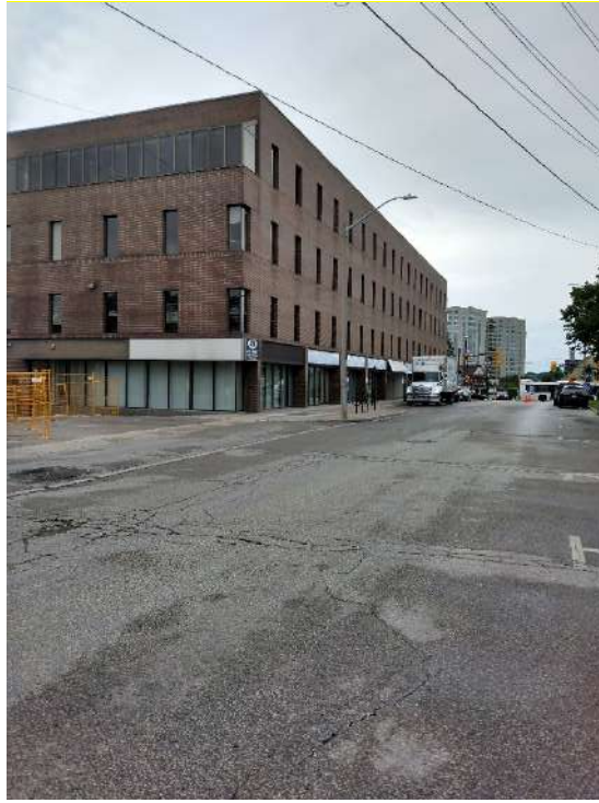
Photograph 1: view of the building, looking southeast along High Street
