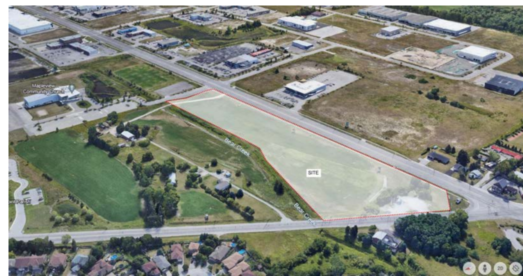
AERIAL VIEW FROM NORTH WEST SIDE
