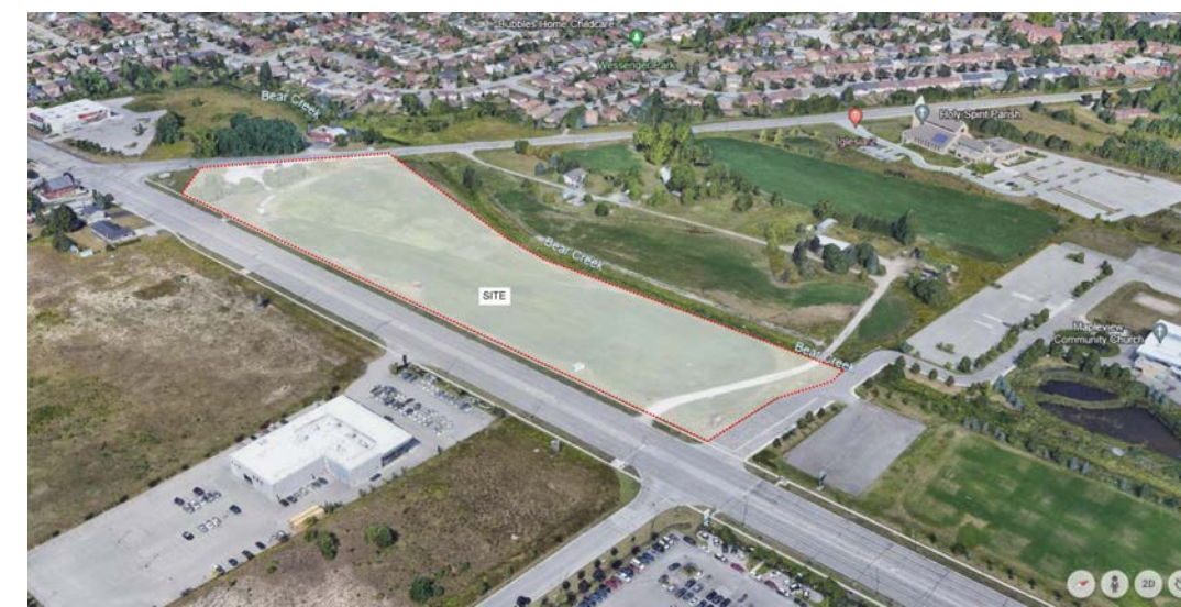
AERIAL VIEW FROM SOUTH EAST SIDE
