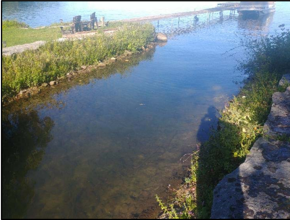
FROM: Right Bank LOOKING: Downstream at Kempenfelt Bay COMMENT: Armourstone lined channel at the mouth
