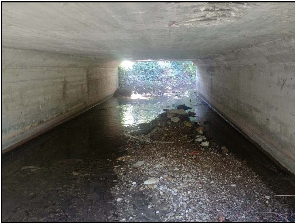
FROM: Centre of creek LOOKING: Upstream through box culvert COMMENT: No distinct low flow channel
