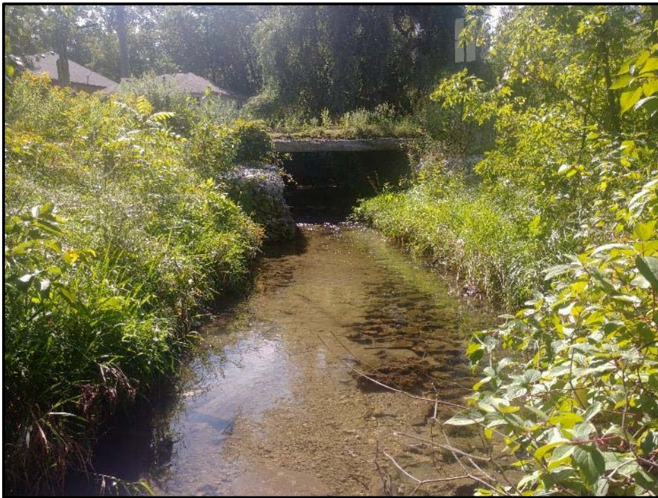
FROM: Centre of creek LOOKING: Upstream at box culvert for Brennan Ave. COMMENT: Gabion leaning, rip rap protecting creek bed
