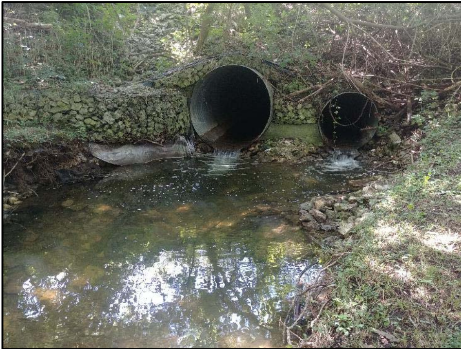
FROM: Centre of creek LOOKING: Upstream towards Hurst Dr culvert COMMENT: Culverts are perched, deep scour pool at outlets
