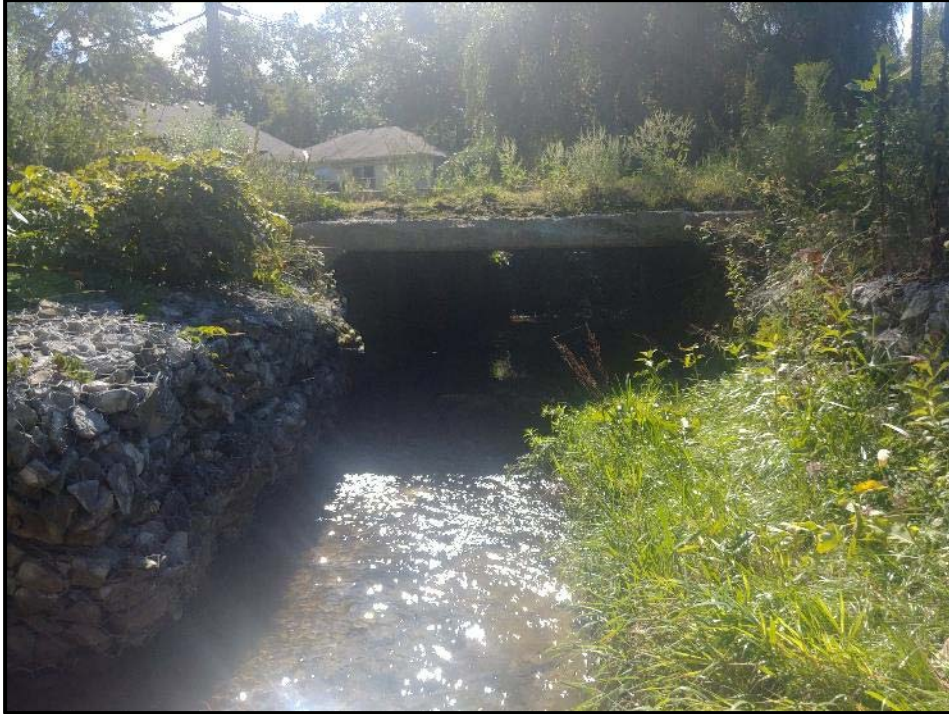
FROM: Centre of creek LOOKING: Upstream at box culvert for Brennan Ave. COMMENT: Gabion visible on right side
