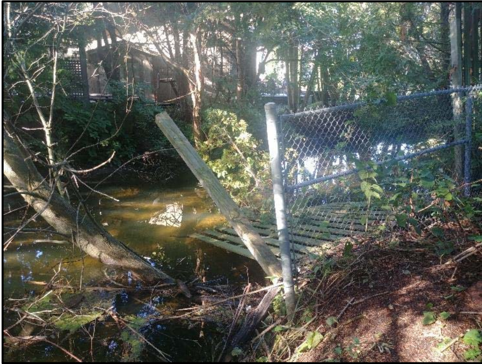
FROM: Right bank LOOKING: Downstream COMMENT: Erosion issues causing fence and tree to fall into creek
