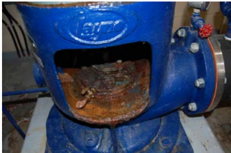
Vertical Turbine Head Assembly
