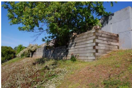
Timber Cribs Planter
