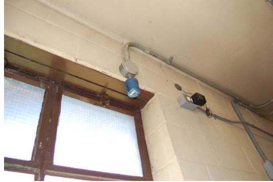
Interior Wall – Pumping Station
