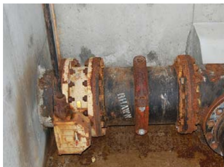
Gate Valve with Gear Operator
