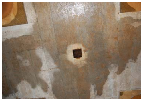
Old Vents Sealed by Wood Plank
