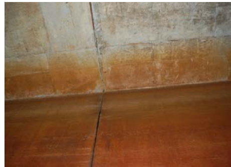
Expansion Joint Sealant (Wall and Roof)
