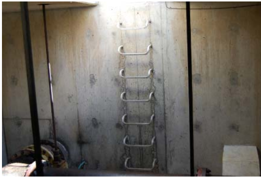
Interior Wall and Ladder Rung -Valve Chamber
