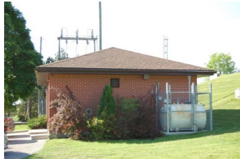
Grading Around the Existing Station
