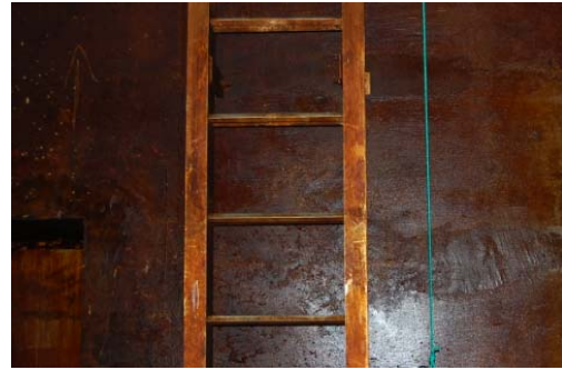
Access Hatch Ladder Rungs
