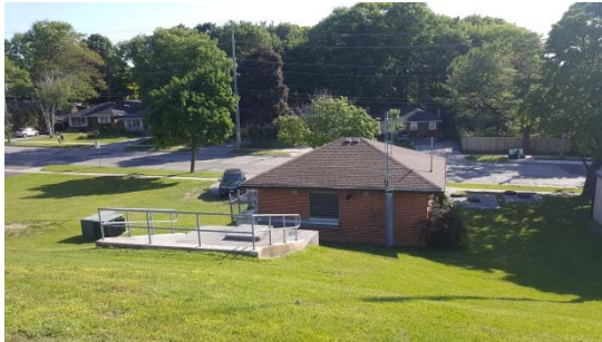
Grading Around the Existing Station
