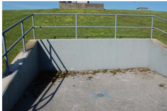
Valve Chamber - Roof Slab, Retaining Wall and Guardrails
