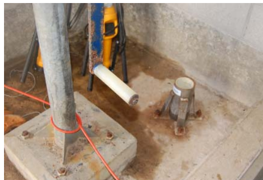
Existing Access Vent House - Floor
