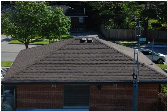
Existing Pumping Station - Roof
