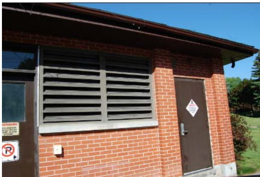
Louver and Chlorination Room - Single Door
