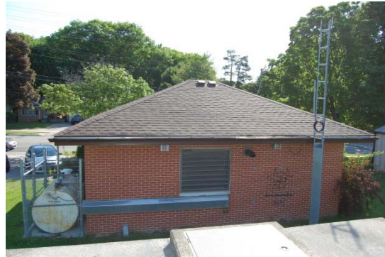
North Wall with Graffiti
