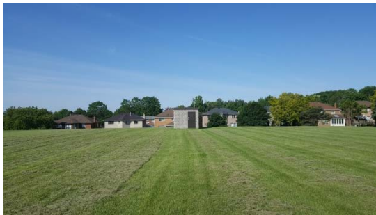
Grading Around the Existing Vent House
