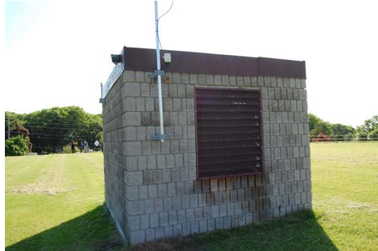
Vent House - Louvre and Grill
