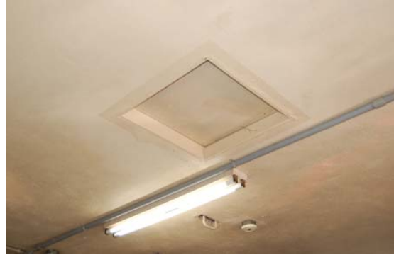
Existing Pumping Station - Access Hatch
