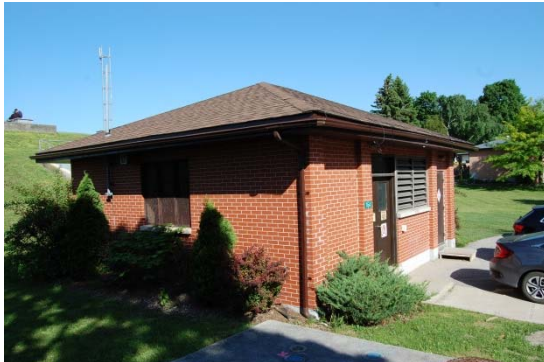
Brick Veneer of Exterior Walls
