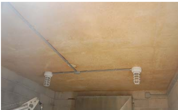
Existing Access Vent House - Ceiling
