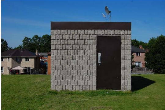
Existing Vent House - West Elevation
