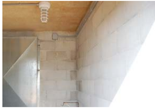
Interior Wall and Ceiling Access/Vent House
