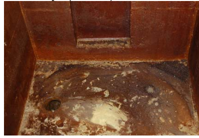
Existing Knockout and Drainage Sump in Cell No.2
