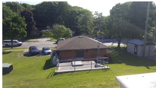
Grading Around the Existing Station
