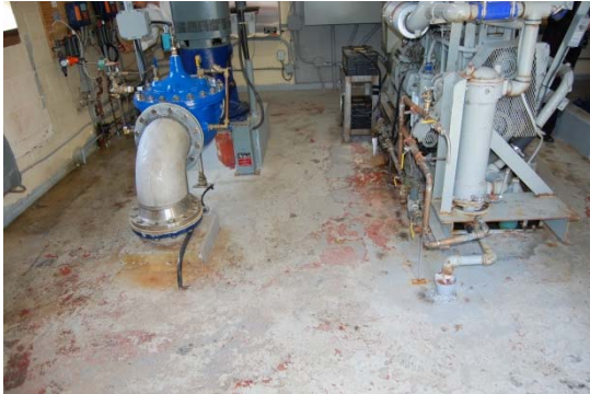
Existing Pumping Station - Interior Floor
