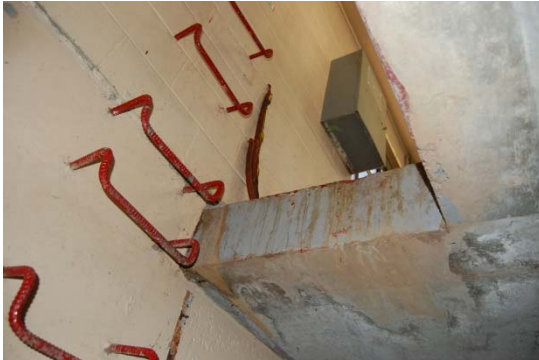
Existing Station Access to Lower Level - Ladder Rungs
