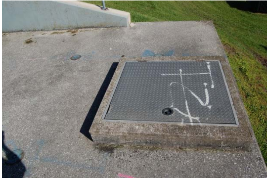
Valve Chamber - Access Hatch
