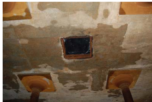
Old Access Hatch Sealed by Metal Plate
