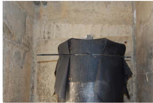
Overflow pipe opening
