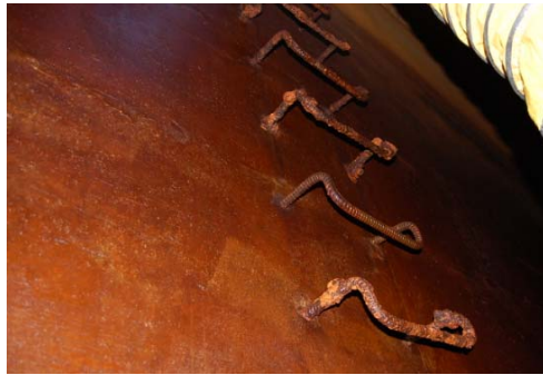
Ex. Manhole Ladder Rungs
