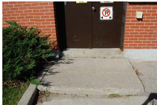
Main Entrance - Double Door
