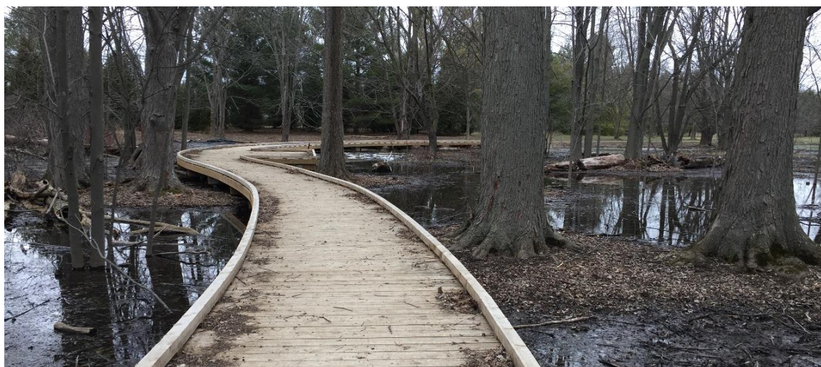
Figure 11 | Low Profile Boardwalk / Elevated Trailbed for Type 4 Trails
