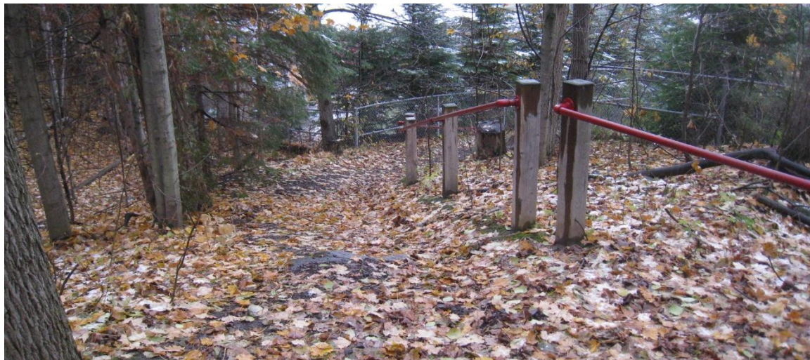
Figure 22 | Crib Stairs (Typical Approach for Type 4 Trails)
