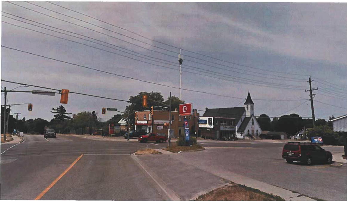
Street view facing west from Penetang Street with tower in place
