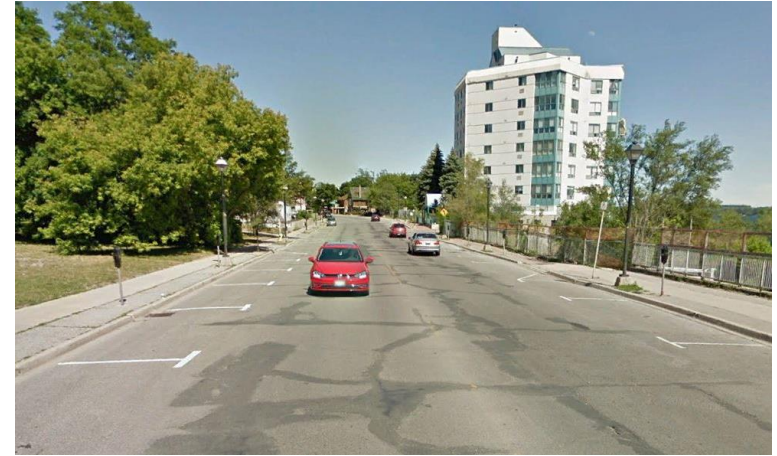
Figure 2c: Dunlop Street East looking east (Site to the left)
