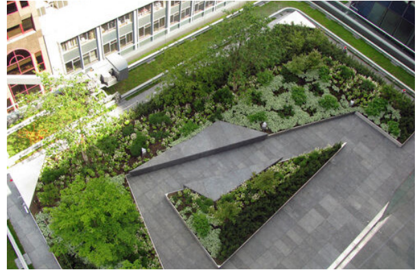
Figure 12.2 Example of a green roof to protect the building from direct solar heat.
