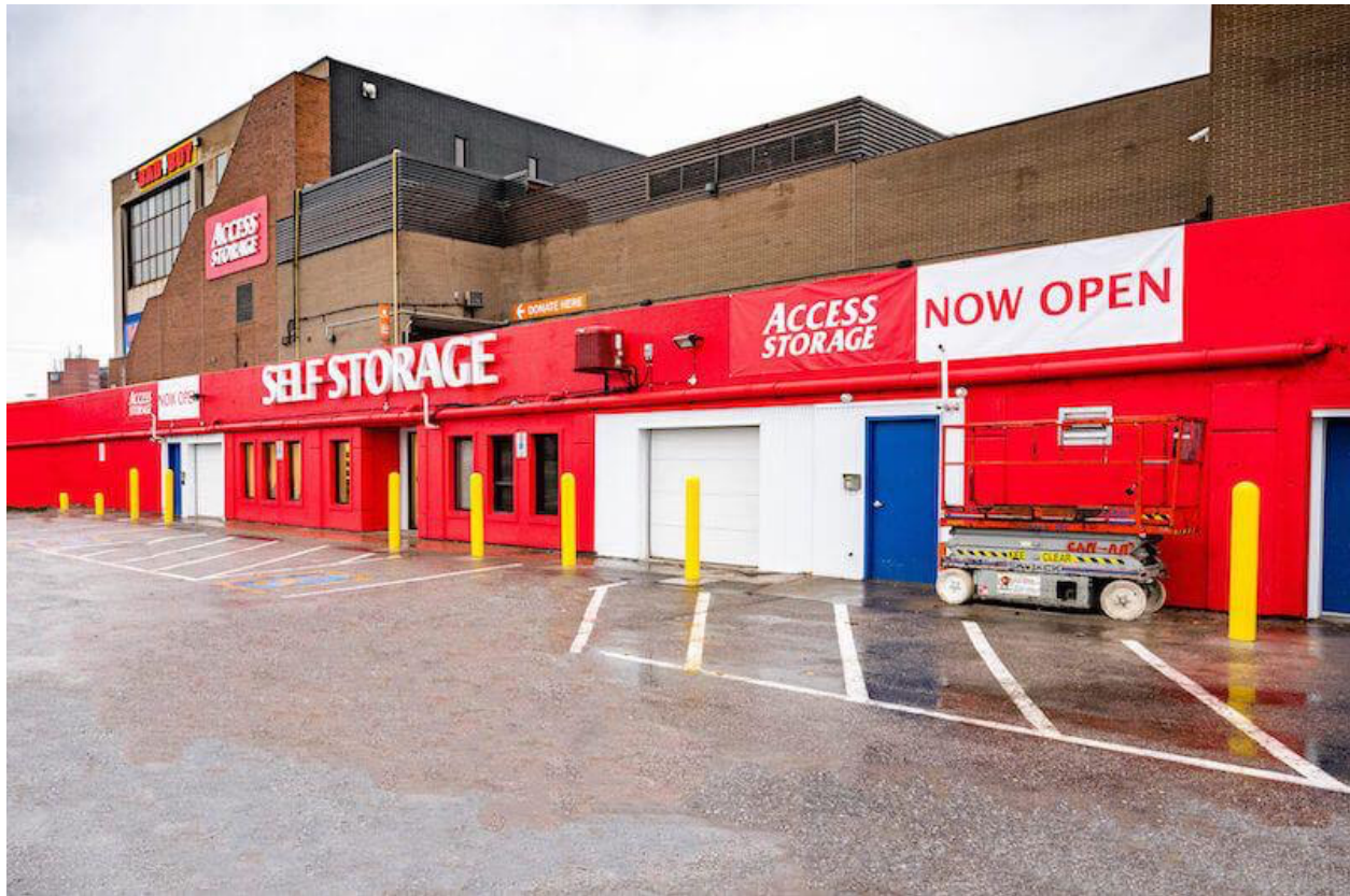
Figure 4: Whitby Shopping Mall (Rear Façade)
