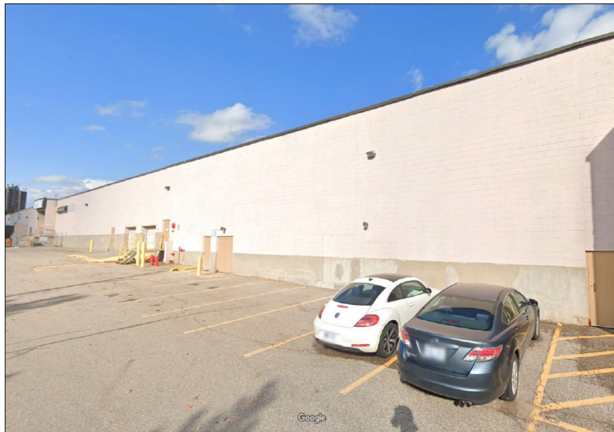
Figure 2: Existing Conditions - Rear of Bayside Mall, and Proposed Self Storage Entrance, South East
