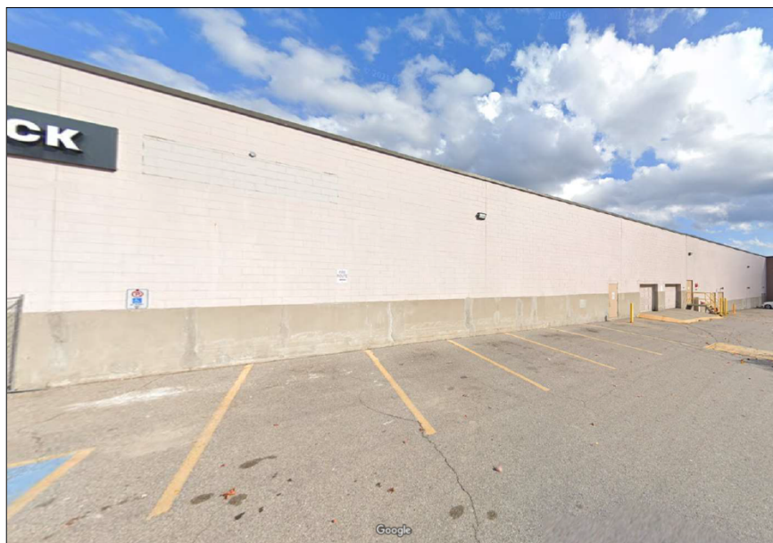
Figure 3: Existing Conditions - Rear of Bayside Mall, and Proposed Self Storage Entrance, North West
