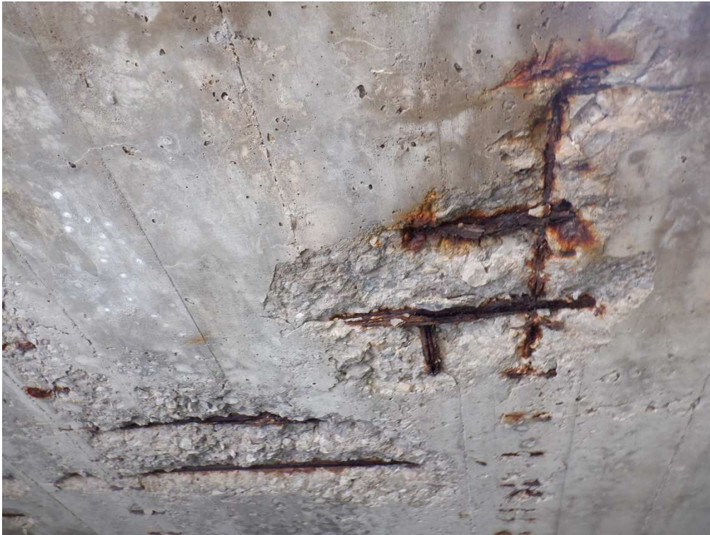
Spall with Exposed, Corroded Rebar in North Exterior Soffit
