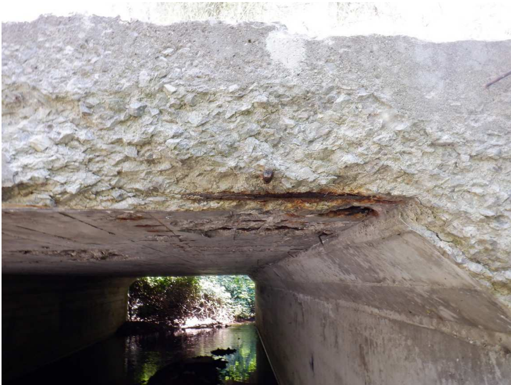
Spall with Exposed, Corroded Rebar at Edge of North Exterior Soffit
