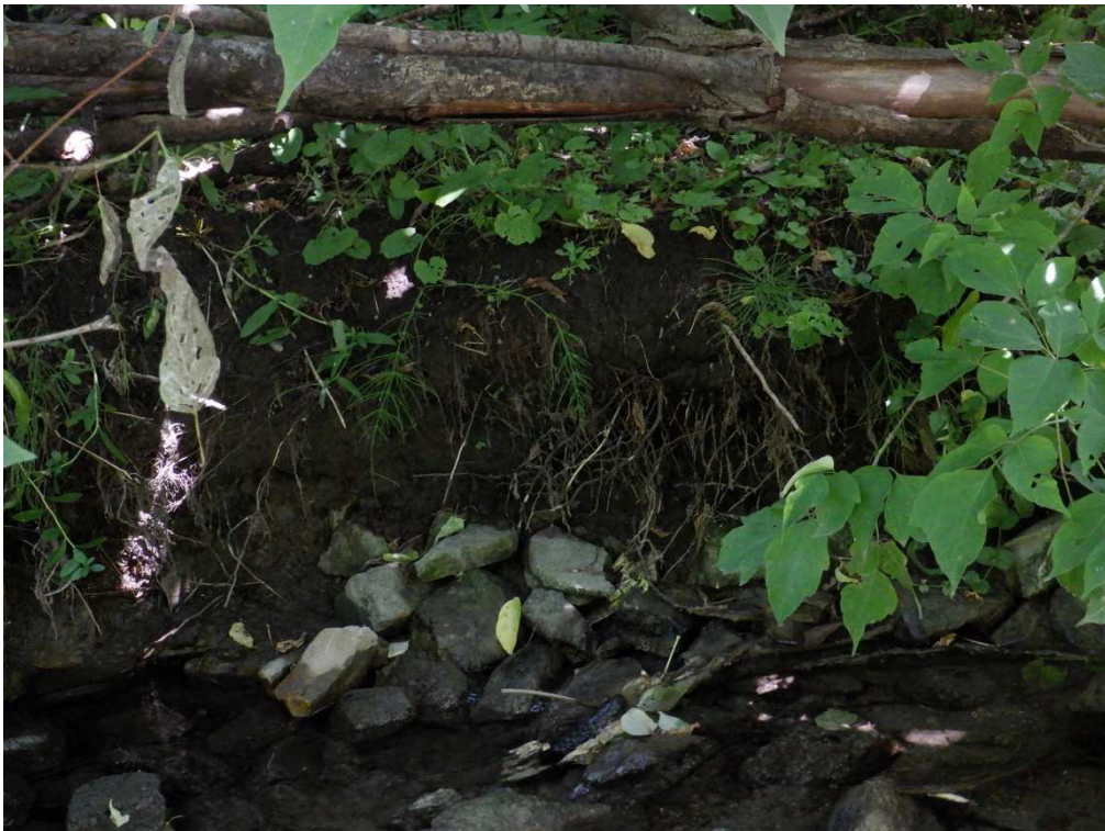
Medium to Severe Erosion of Southeast Embankment
