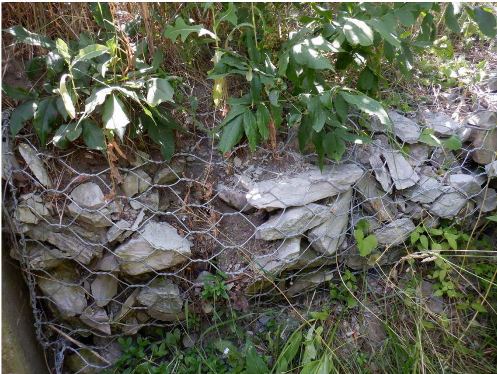
Loss of Stone from Gabions
