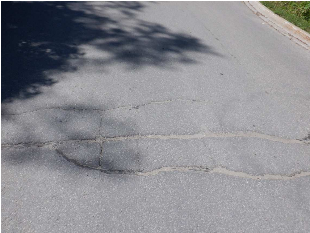
Wide Cracks in Southeast Approach
