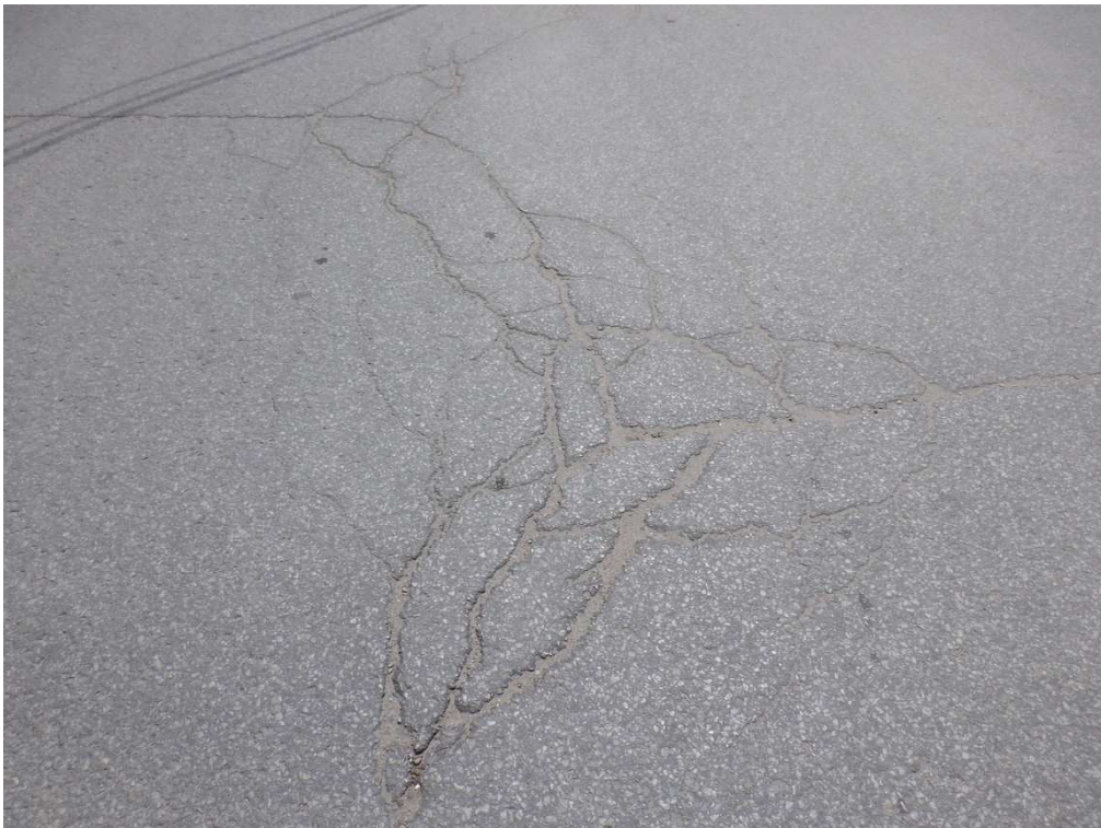
Wide Map Cracks in Asphalt Wearing Surface
