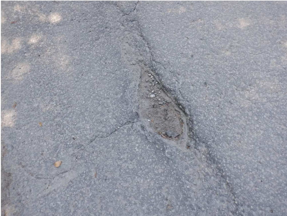
Pothole in Northwest Approach Asphalt Wearing Surface
