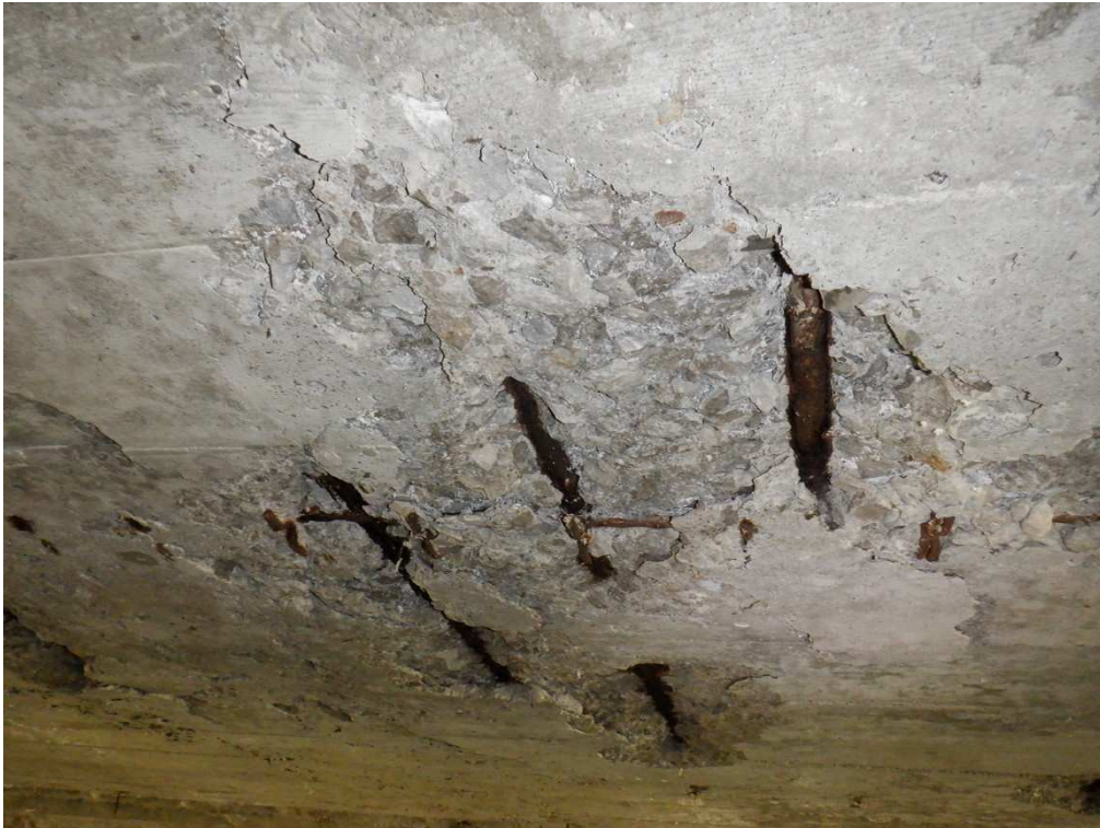
Delaminations and Spalls with Exposed, Corroded Rebar in Interior Soffit
