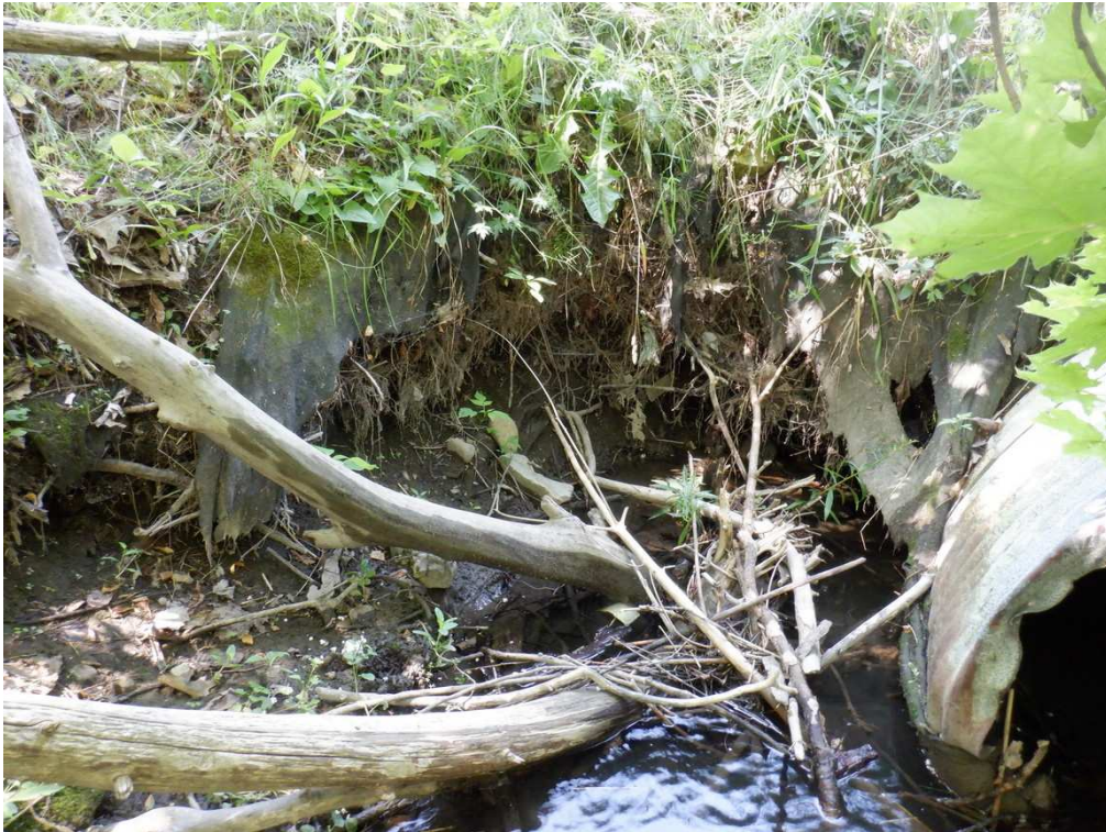
Medium to Severe Erosion of Northwest Embankment
