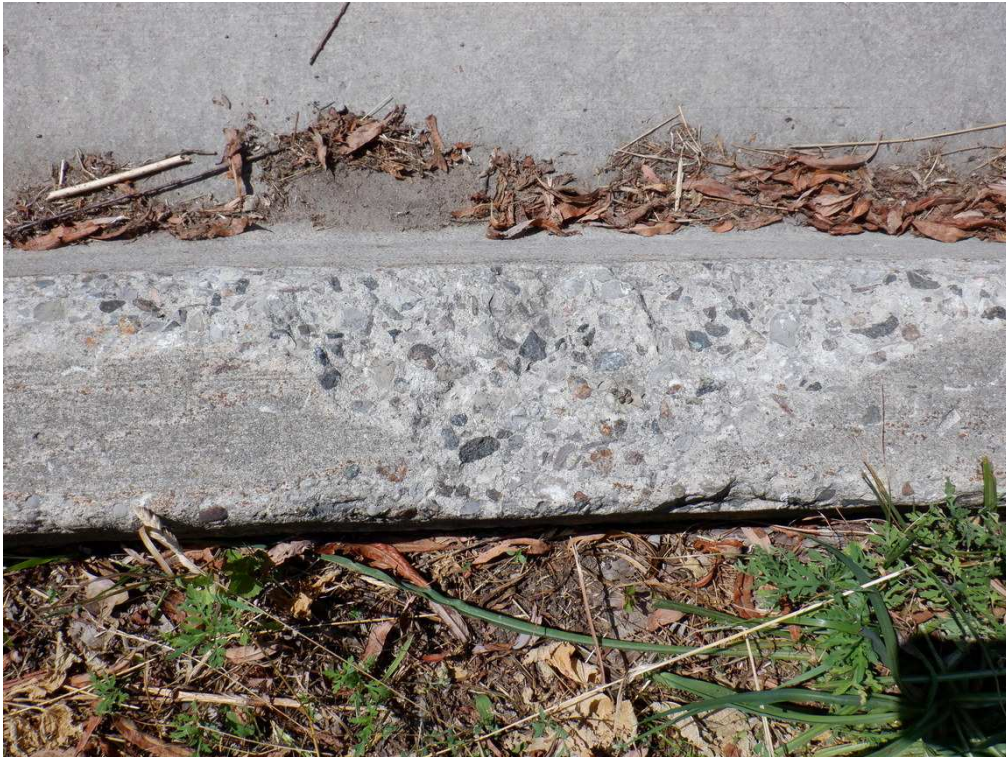
Medium to Severe Scaling of Curb
