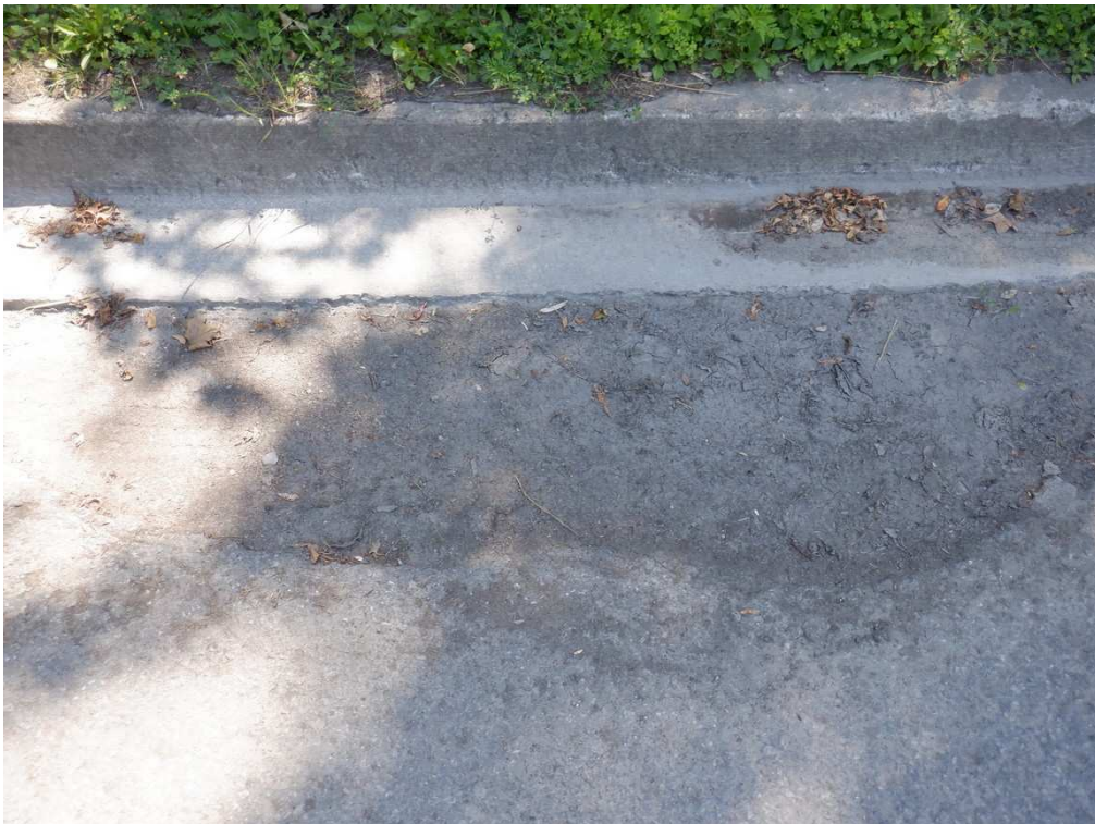
Settlement of Edge Asphalt along West Edge
