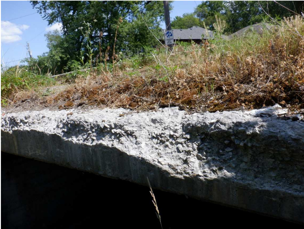
Large Spall and Severe Scaling of North Fascia
