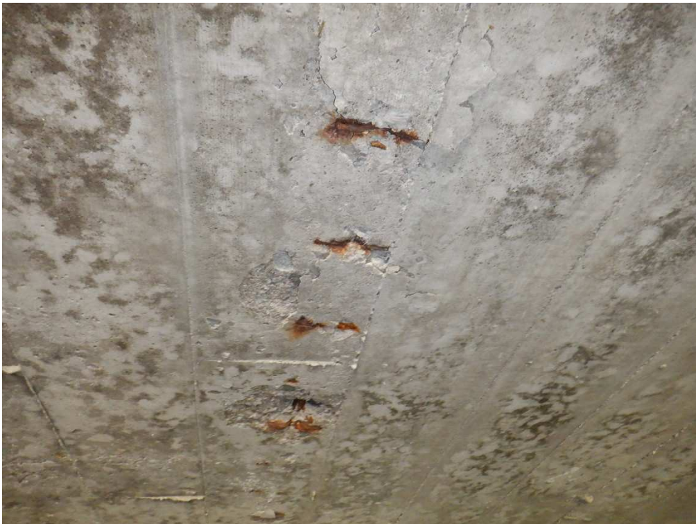
Delaminations and Small Spalls with Exposed, Corroded Rebar in Interior Soffit
