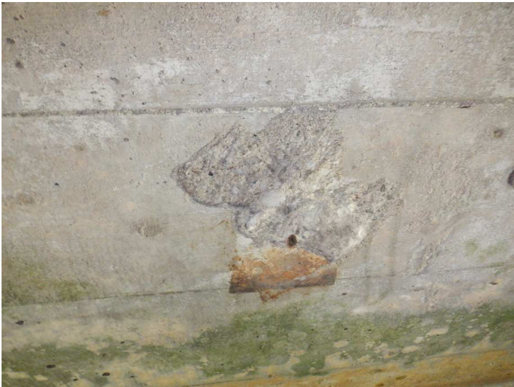
Spall in East Wall
