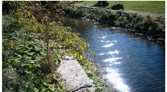
Photo 4. Reach 1 along Whiskey Creek with harden edges and adjacent residential yard (September 23, 2020).
