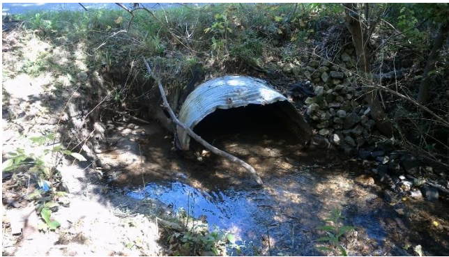
Photo 9. Existing culvert under The Boulevard (September 23, 2020).
