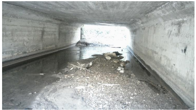
Photo 10. Existing culvert under Brennan Avenue, note lack of bird nests (September 23, 2020).
