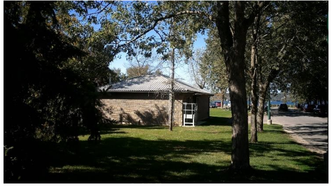
Photo 8. Existing structure and entrance for Minet's Point Park, possible relocation September 23, 2020).
