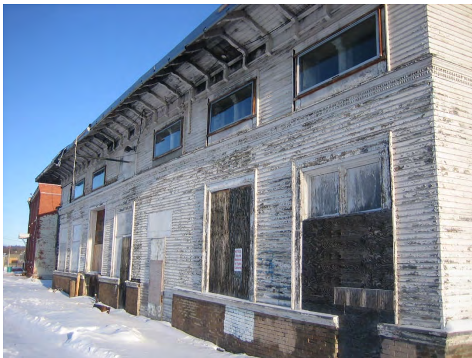
Photo 16 – Exterior of the south side of the former restaurant/freight storage building looking northwest. Note peeling paint.
