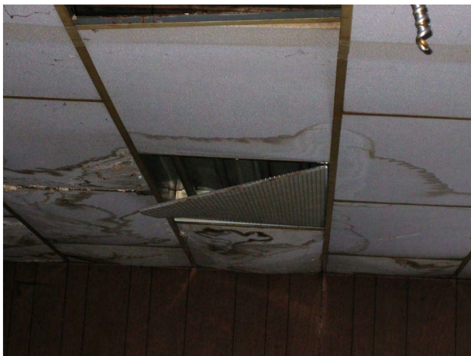
Photo 18 – Water damage on the ceiling in the former passenger station.
