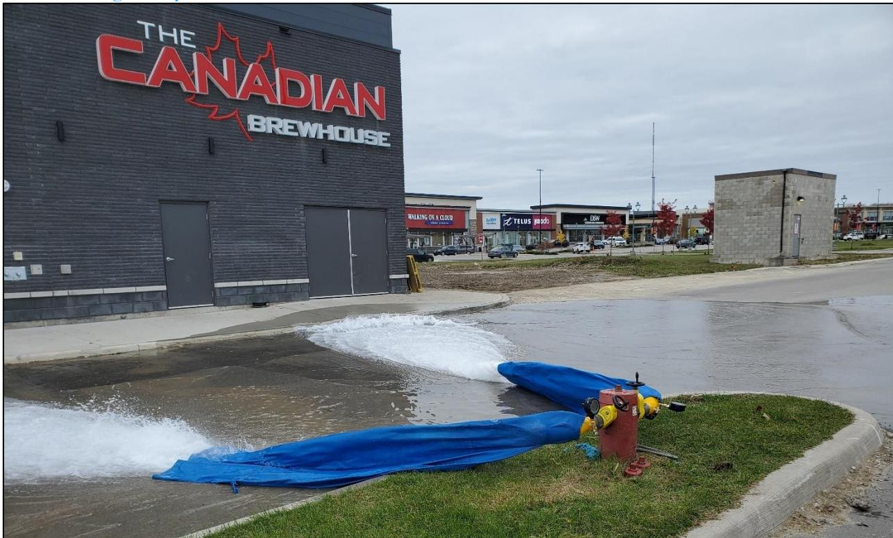
Figure 11: Hydrant flow test at flow hydrant F2 (HY39) – SW parking lot at S Village Way and Live Eight Way, 1st S
