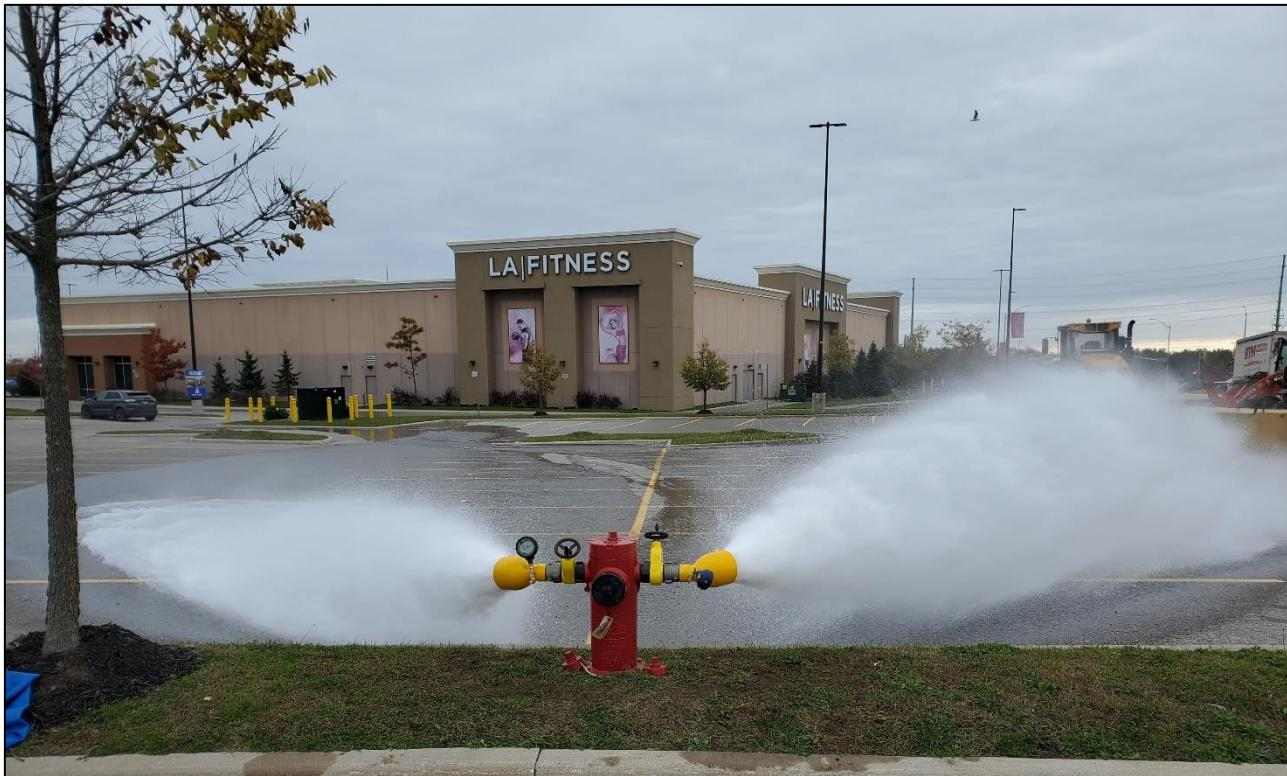
Figure 10: Hydrant flow test at flow hydrant F1 (HY29) – NW parking lot at S Village Way and Live Eight Way, 1st N
