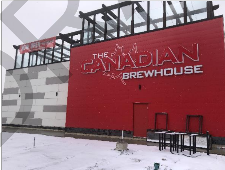
Photo 6 – Southern elevation of the Site Building, looking northwest.
