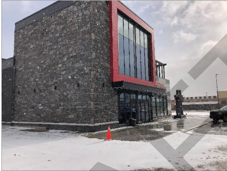
Photo 7 – Western elevation of the Site Building, looking southeast.
