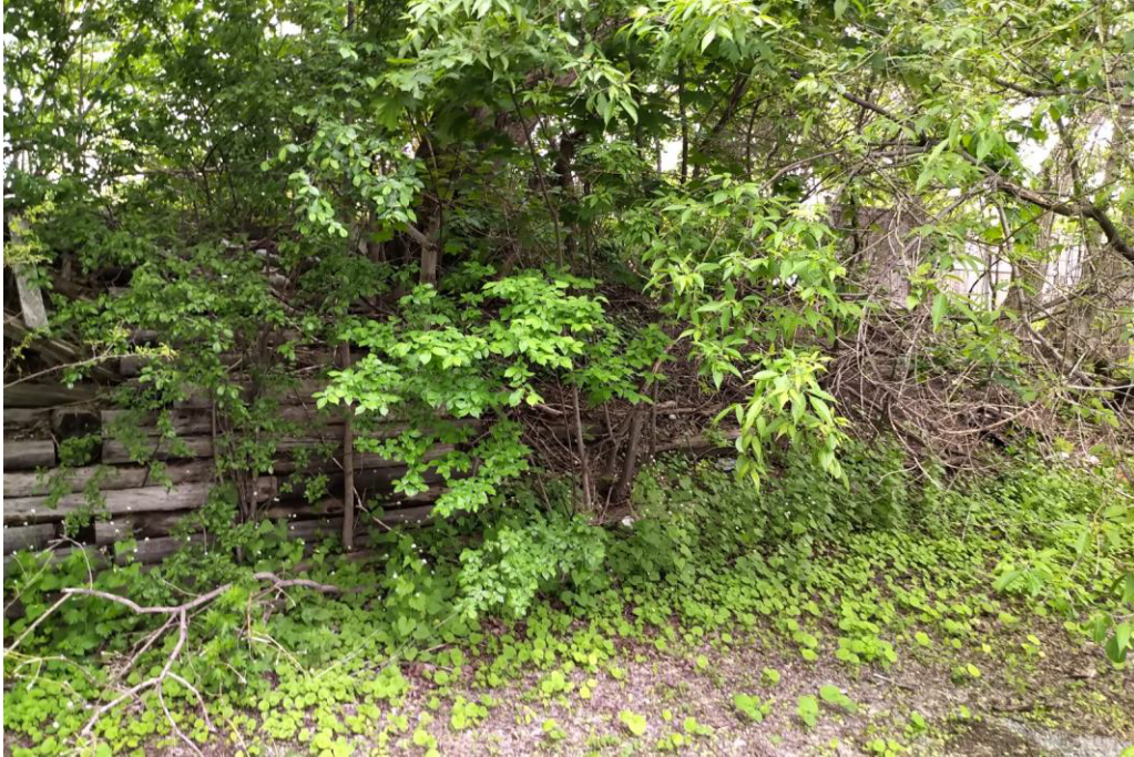
Photograph No. 3 – Northeast facing view of the retaining wall in the eastern portion of the Site.
