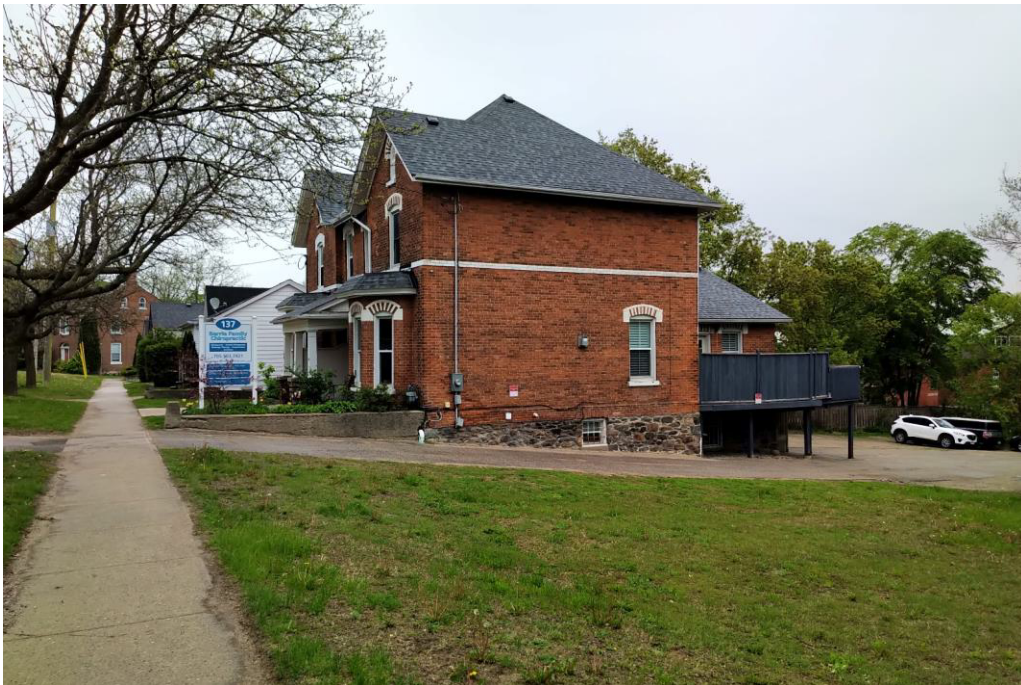
Photograph No. 10 – East facing view of the east adjoining property (137 Collier Street).
