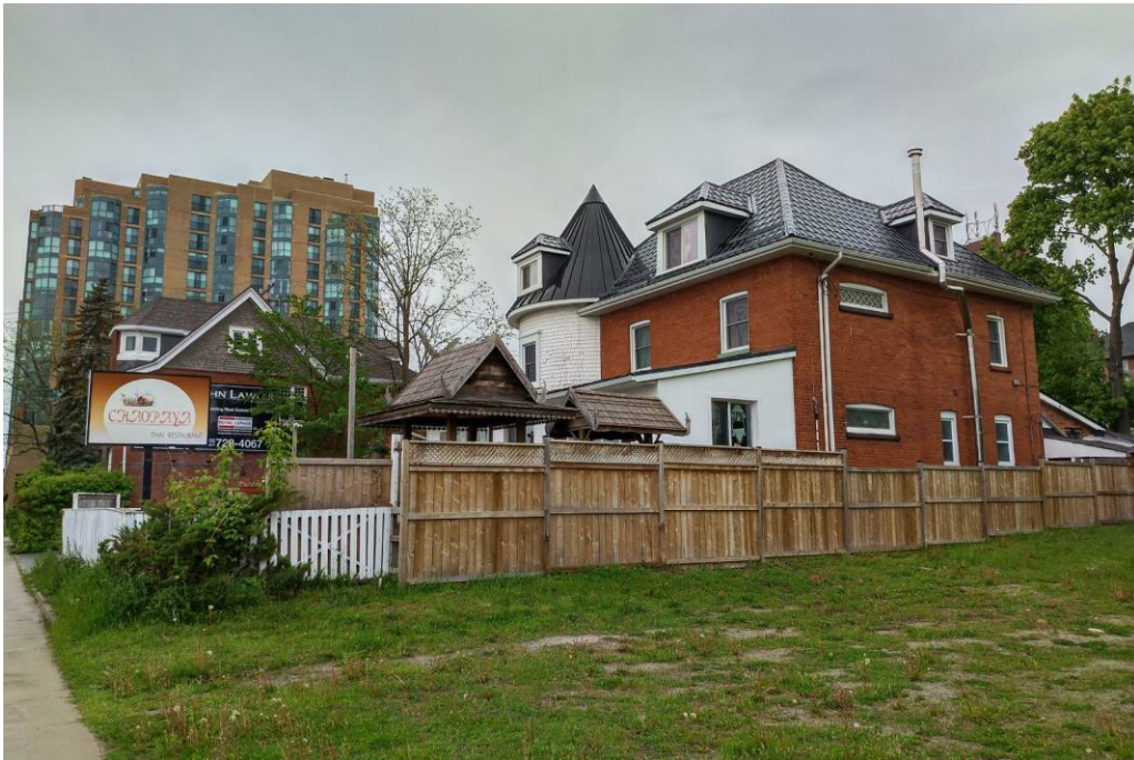
Photograph No. 7 – Northwest facing view of the west adjoining property (168 Dunlop Street East) where TSSA records identified underground storage tanks.
