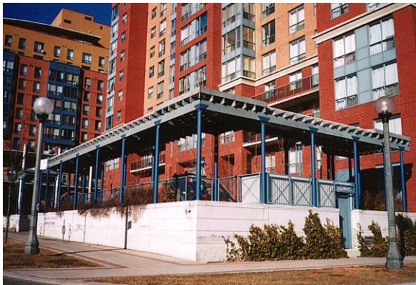
Image 10: Examples of Wind Control Measures at Building Corners and Amenity Areas
