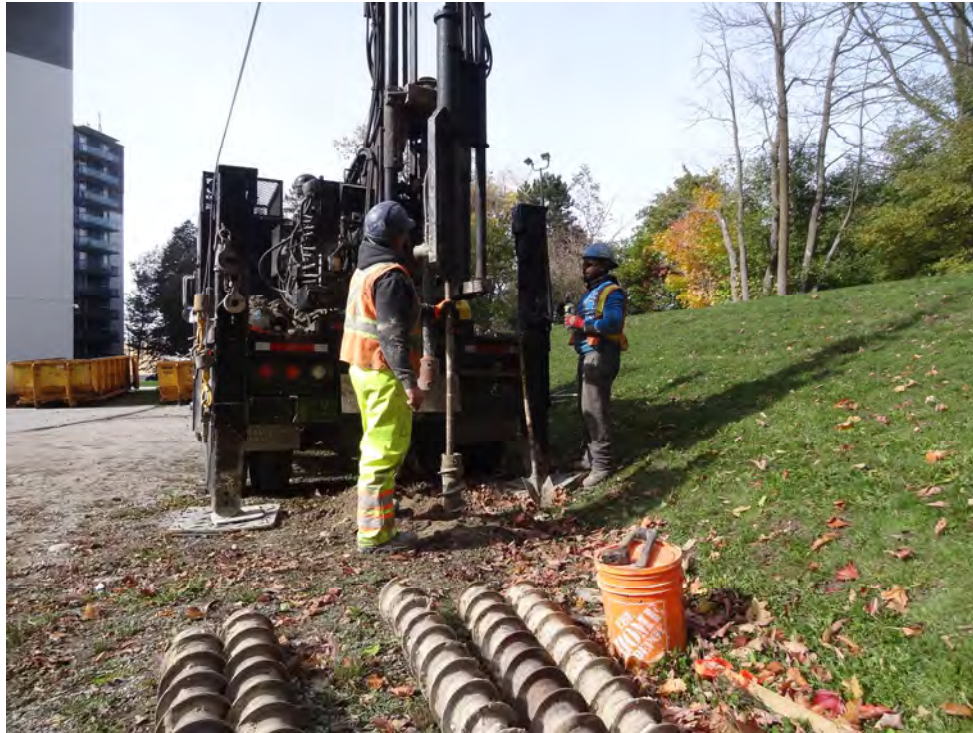
Photograph No. 7 – Drilling at Borehole BH5 Location, West View
