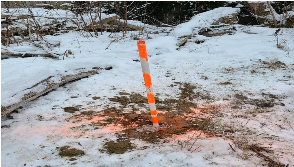
Piezometer stand pipe installed at Borehole No. 1
