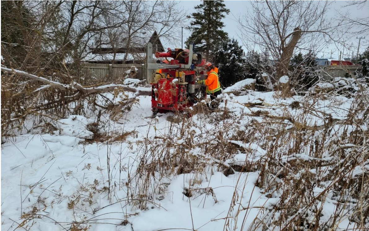
Drilling Borehole No. 4
