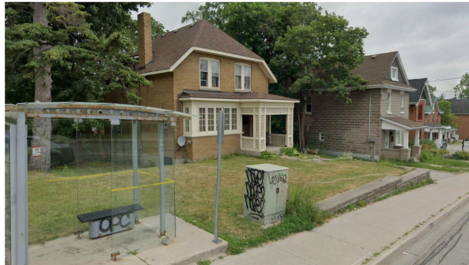
219 Bayfield Street, looking south east
