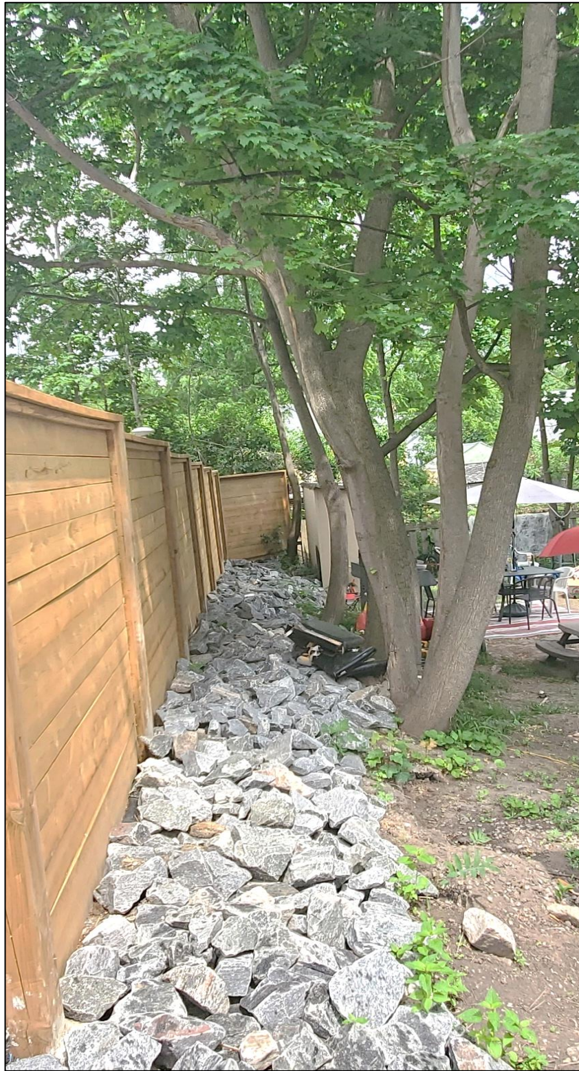
Photo D: Tree D, E, F, G (Norway Maple), located onto residential property 215 Bayfield Street. Wooden fence and large stone (3m landscape buffer; Site Plan) constructed above the tree's root systems. Evidences of deadwood, epicormic branching and leans. Photo facing north.
