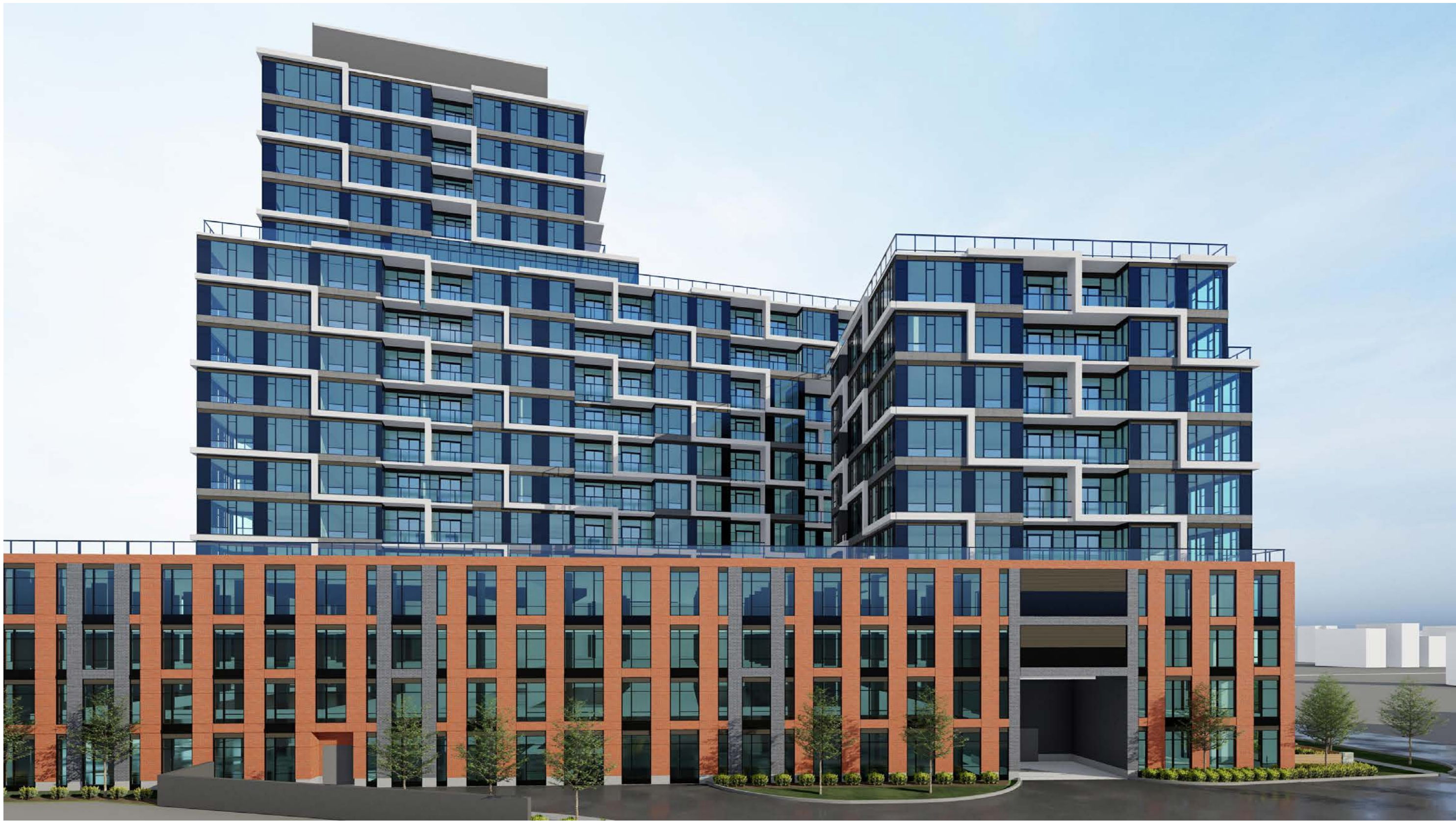
SOUTH OF CONDO LOOKING NORTH 2 A703
