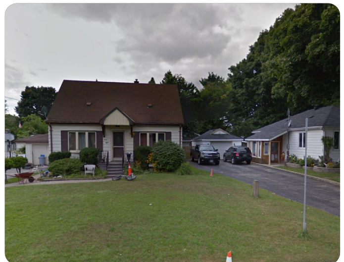
Figure 6: Residential Homes on Marcus Street - Google Street View
