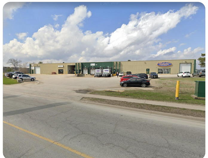
Figure 11: Industrial building on Tiffin Street - Google Street View
