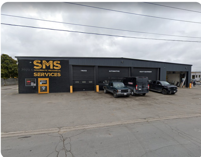
Figure 10: Industrial building on Brock Street - Google Street View
