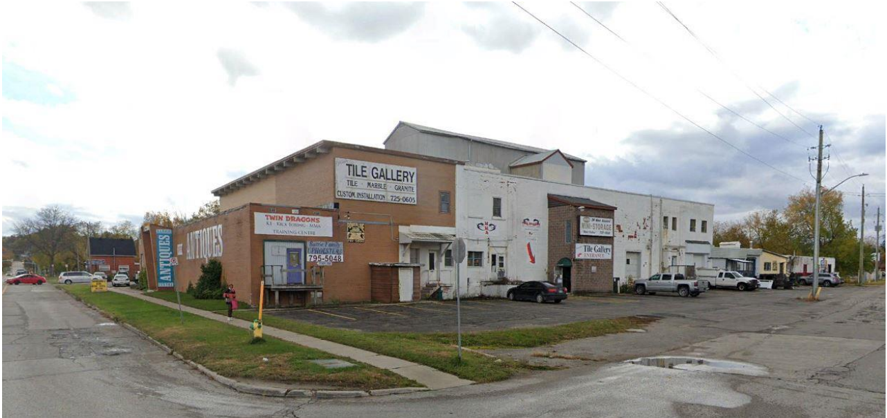
272 Innisfil Street proposed Development Site Looking Southwest from Innisfil Street
